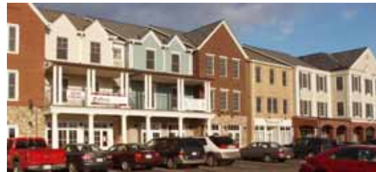
Located next to the historic Winterham building, this building is the current home to:
