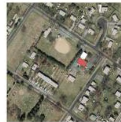
Current Municipal Building Renovation/Expansion
