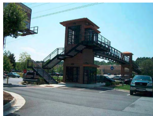
Bicycle & Pedestrian Bridge Over Roadway (City of Lynchburg)
