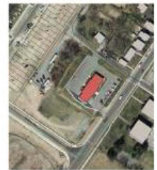
Former BB&T Bank Building Renovation
