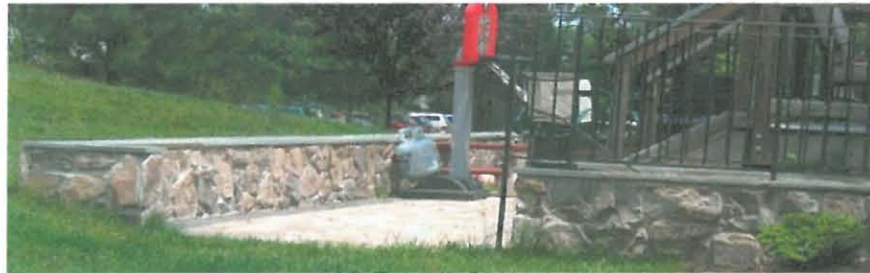
Stone Retaining Wall
