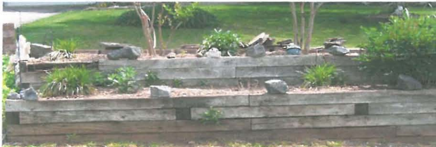
Wood Retaining Wall
