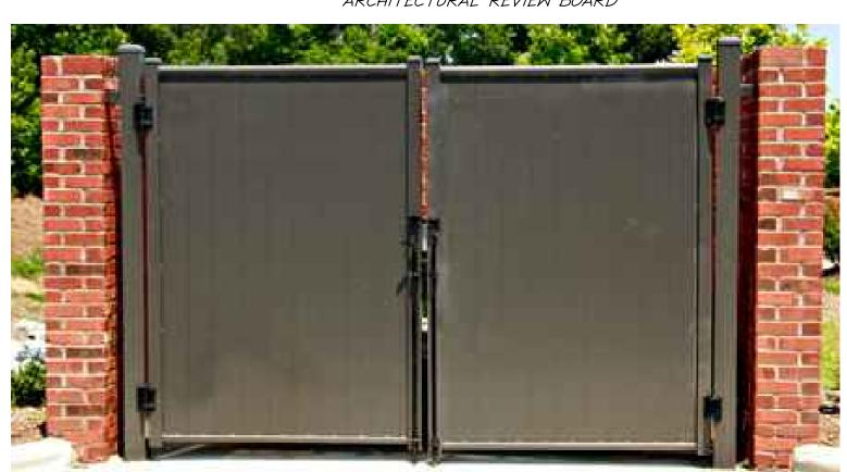
DUMPSTER GATE DETAIL MATERIAL TO BE PVC OR ALUMINUM LOUVERS
