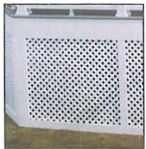
WHITE PVC LATTICE AROUND PERIMETER BELOW BOTH DECKS
