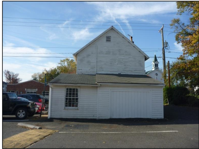
Rear View of Ex. Building
