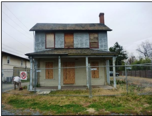
Photo 1 - Front View of Ex. Building
