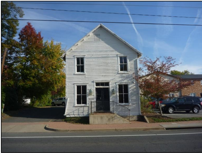
Front View of Ex. Building
