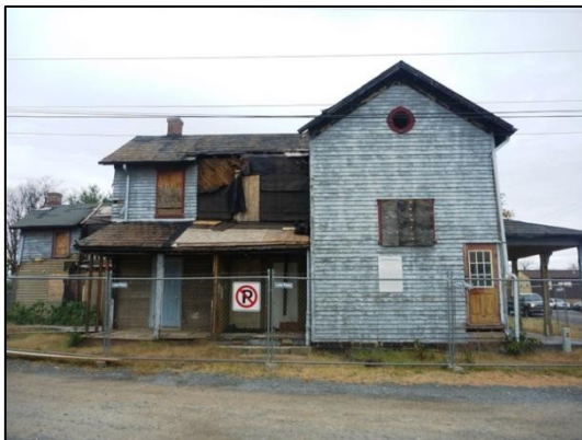
Photo 3 -View of left side of building
