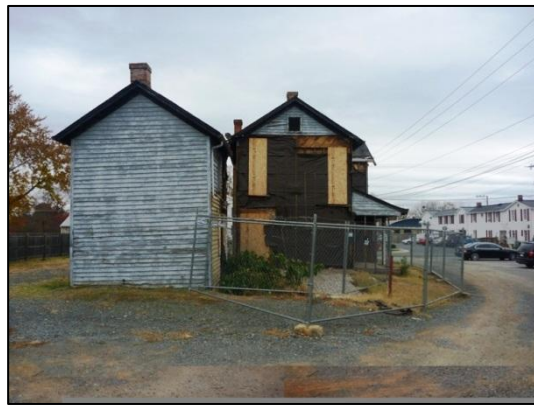
Photo 2- Rear View of Ex. Building
