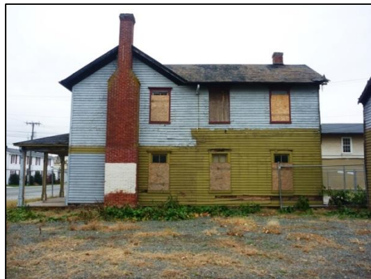
Photo 4- View of right side of building
