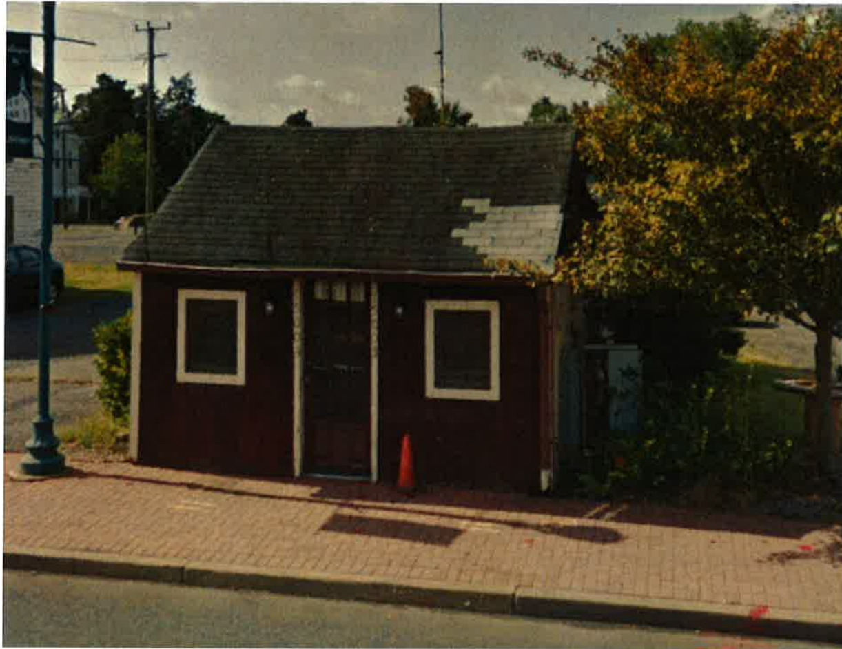
Photographs of 15003 Washington Street - Structure I
