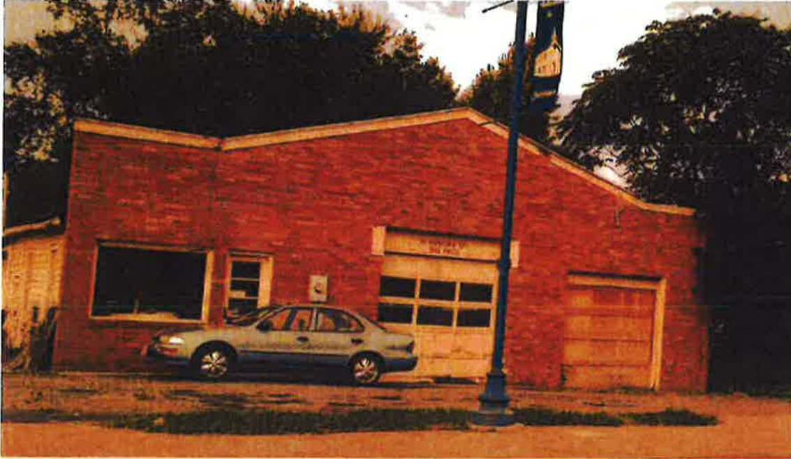
Structure A – Front:
