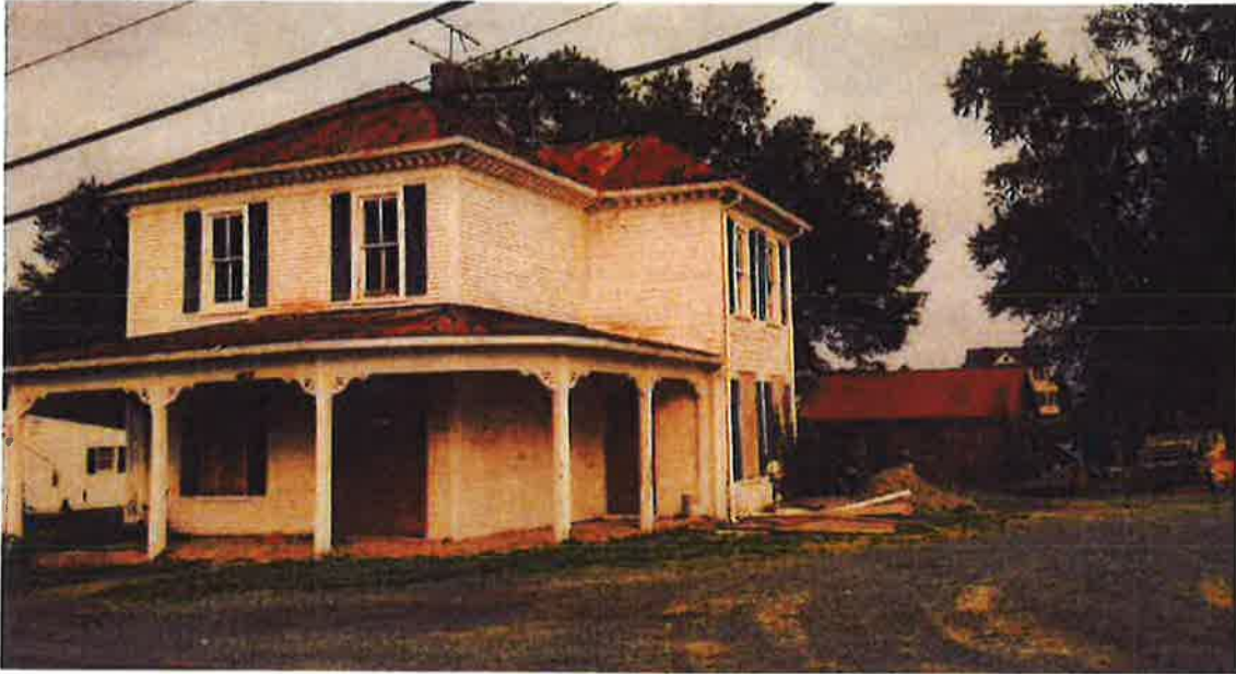
Photographs of 6706 Jefferson - Structure F
