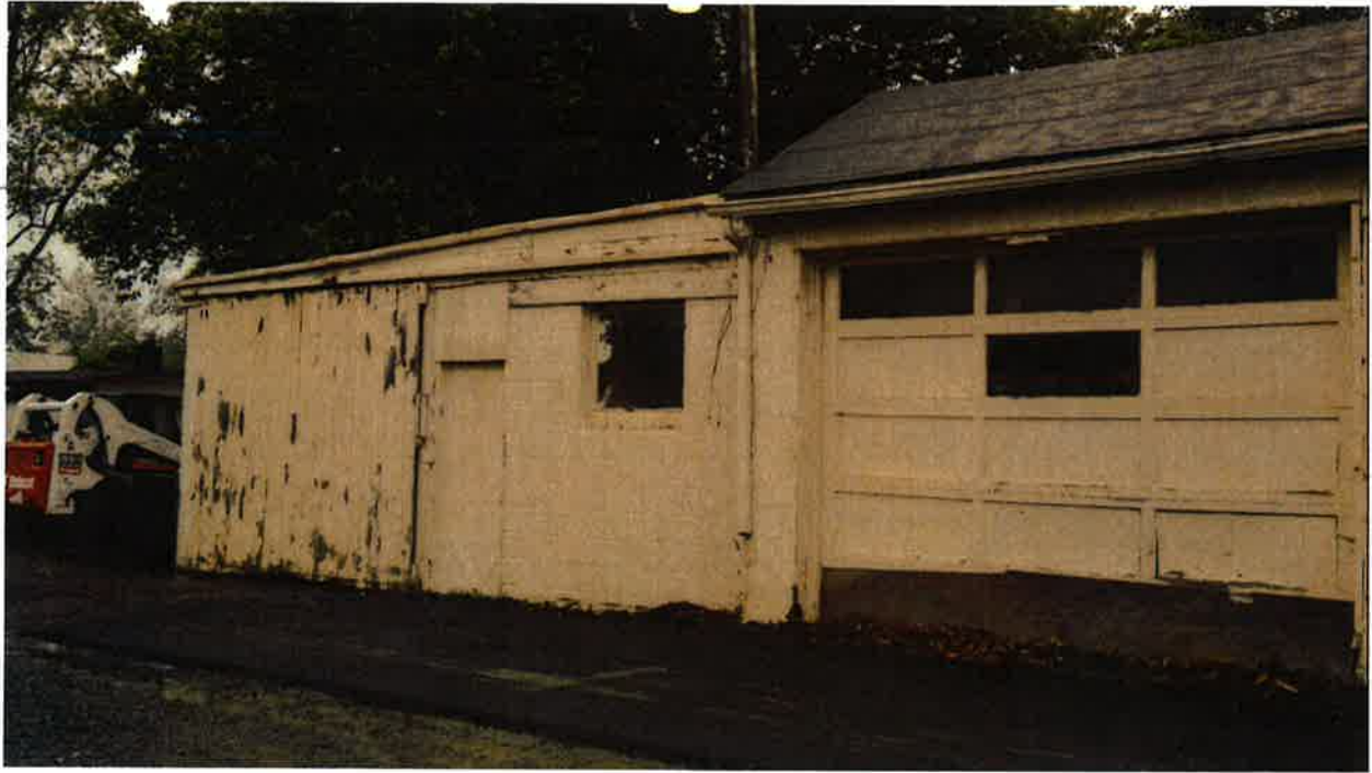
Structure A – Side:
