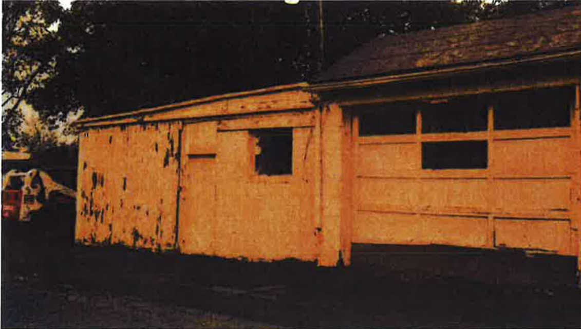
Structure A – Side:
