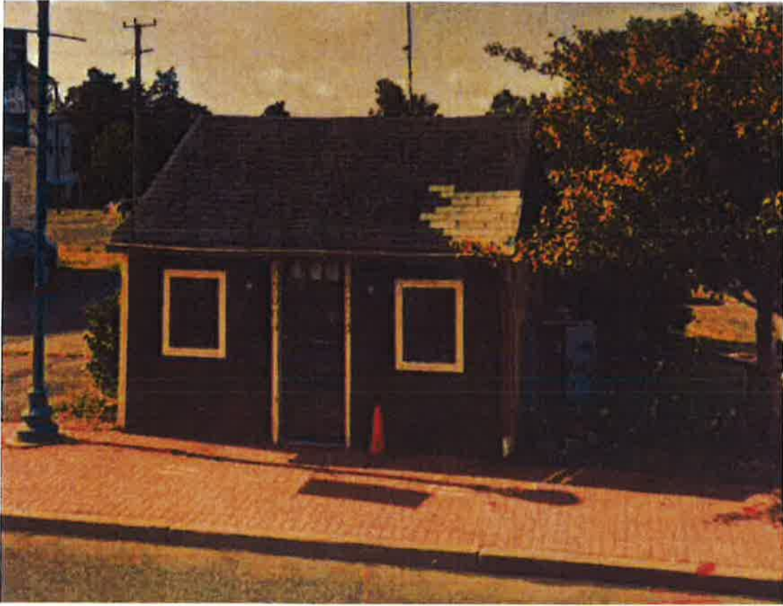
Photographs of 15003 Washington Street - Structure I
