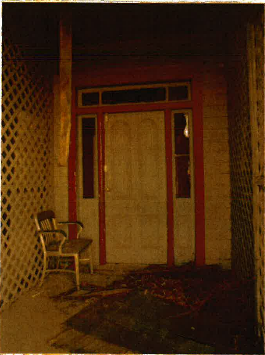
Photo #3: Broken windows at front door
