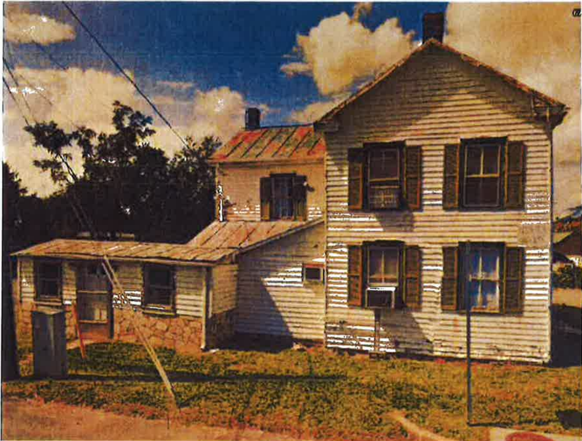
Photographs of 15001 Washington Street – Structure H
