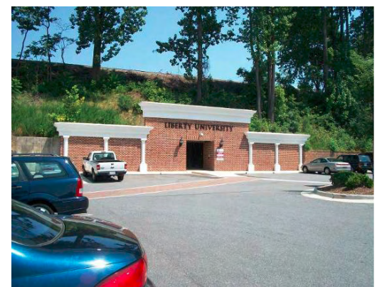
Bicycle & Pedestrian Tunnel Under Railroad (Liberty University)
