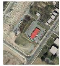
Former BB&T Bank Building Renovation
