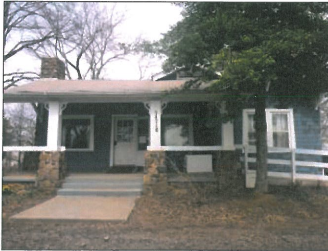
Photo 1 – View of front of subject house
