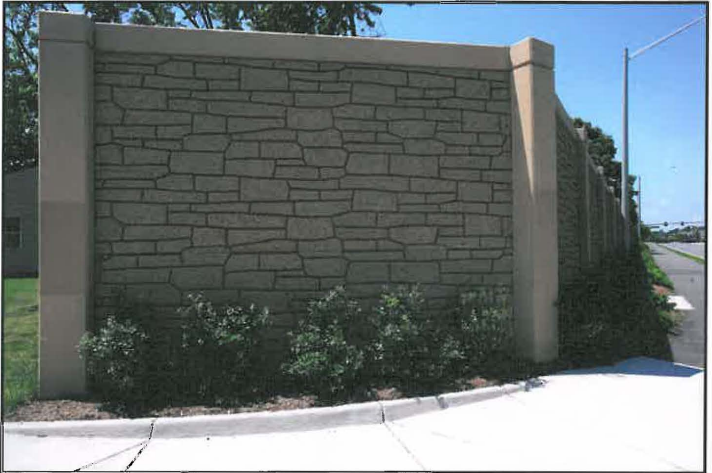
Roadway side-SanDiego DryStack
