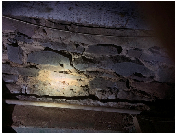
Condition of original foundation wall at basement stairs
