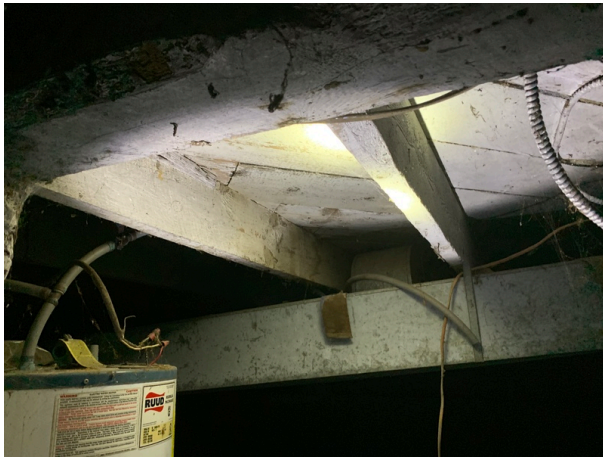
Wood joist viewed from underside of floor in basement.
