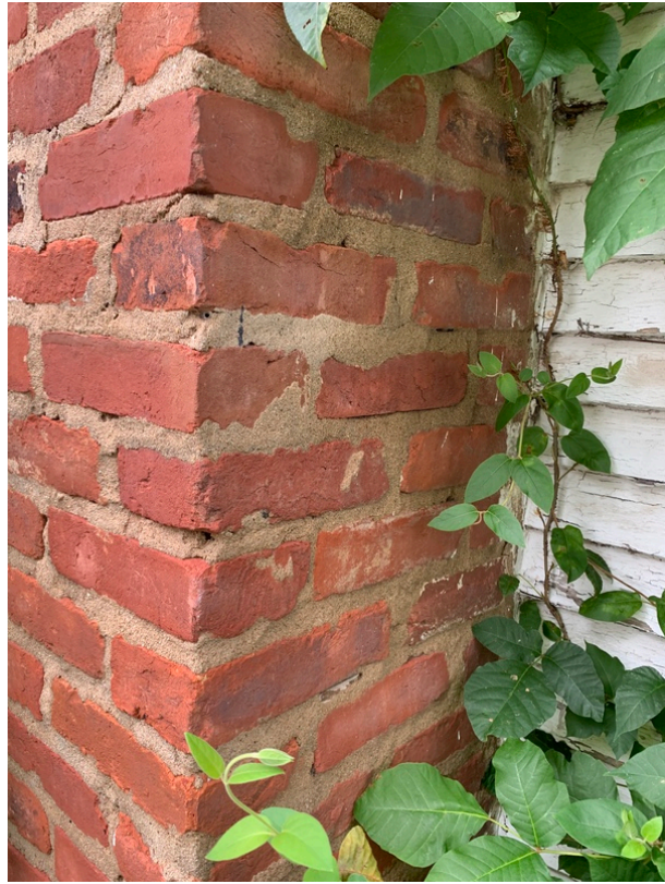
Chimney at addition
