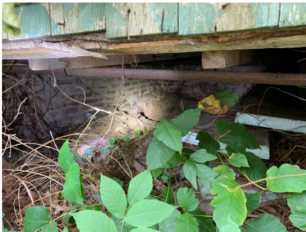
Brick Foundation on Addition
