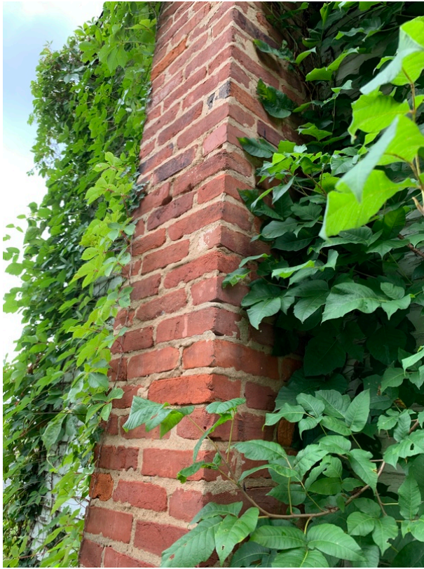
Chimney at addition
