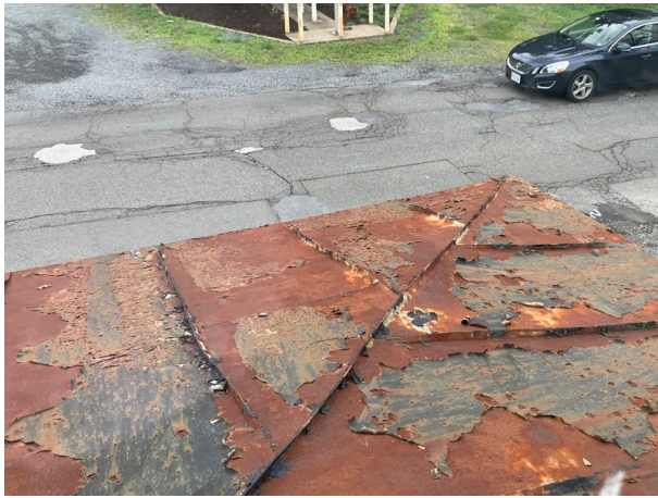
Close up of porch roof
