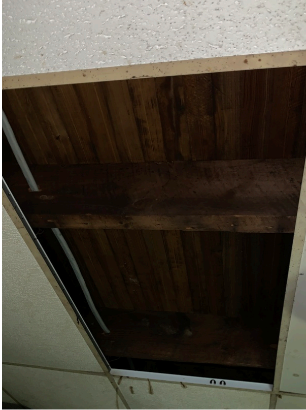
Wood joist viewed from interior hole in ceiling
