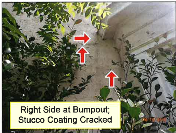
2.0 SIDING / WALL CLADDING (Picture 3)
