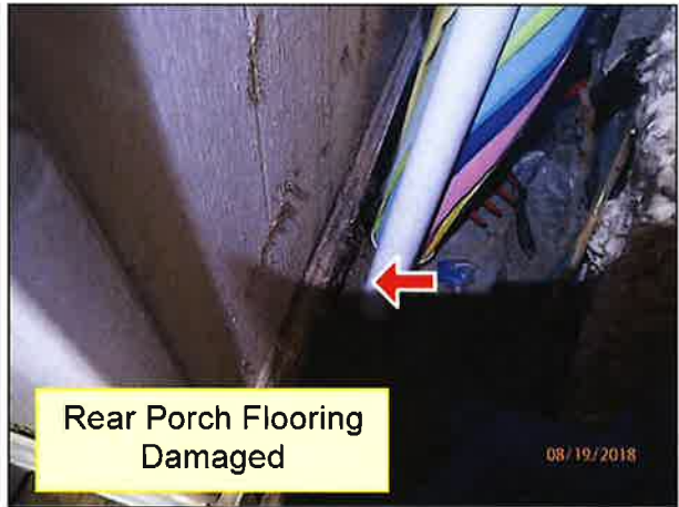
2.6 REAR PORCH (Picture 3)
