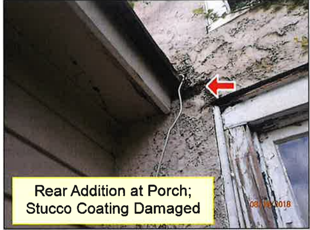
2.0 SIDING / WALL CLADDING (Picture 2)
