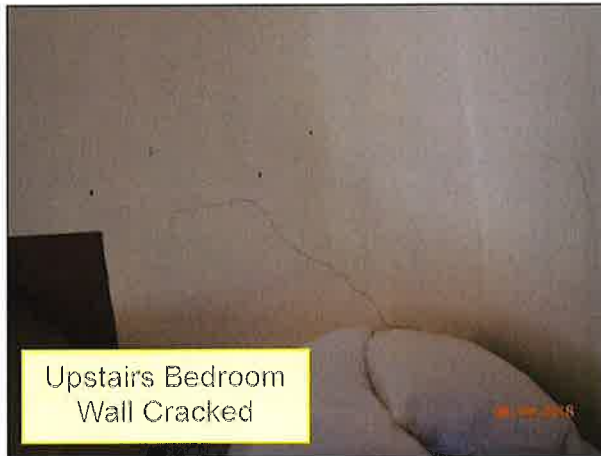
4.1 WALLS / STRUCTURE (Picture 4)
