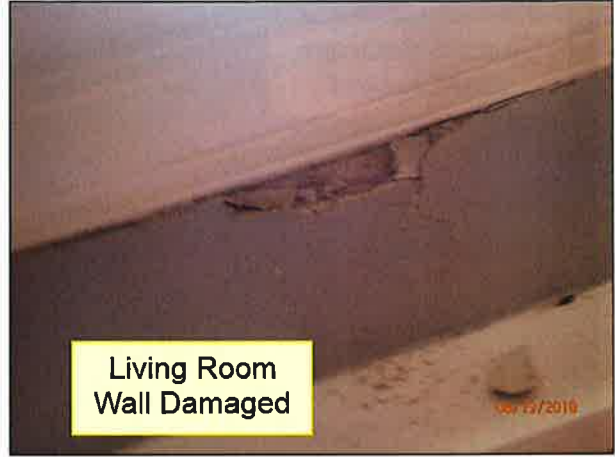
4.1 WALLS / STRUCTURE (Picture 13)
