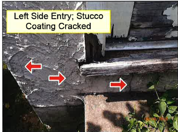
2.0 SIDING / WALL CLADDING (Picture 6)
