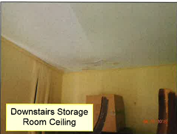
4.0 CEILINGS / STRUCTURE (Picture 13)
