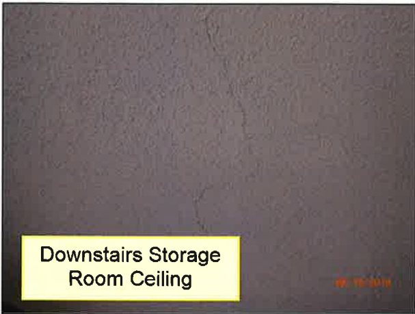
4.0 CEILINGS / STRUCTURE (Picture 11)
