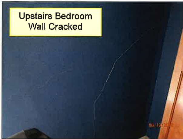
4.1 WALLS / STRUCTURE (Picture 6)
