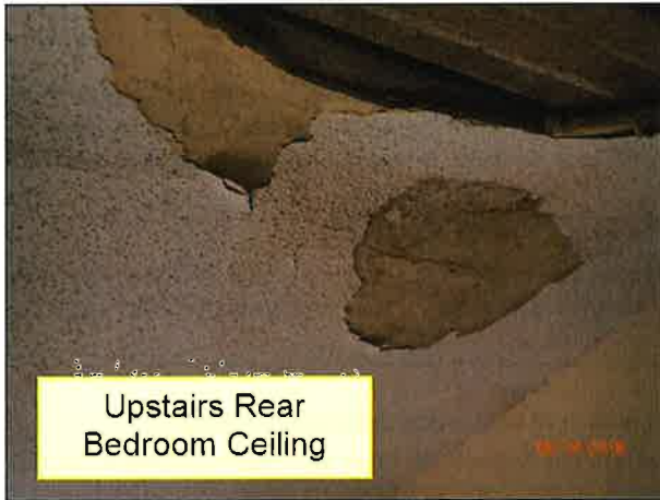
4.0 CEILINGS / STRUCTURE (Picture 5)
