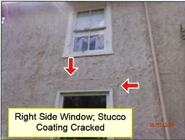
2.0 SIDING / WALL CLADDING (Picture 9)
