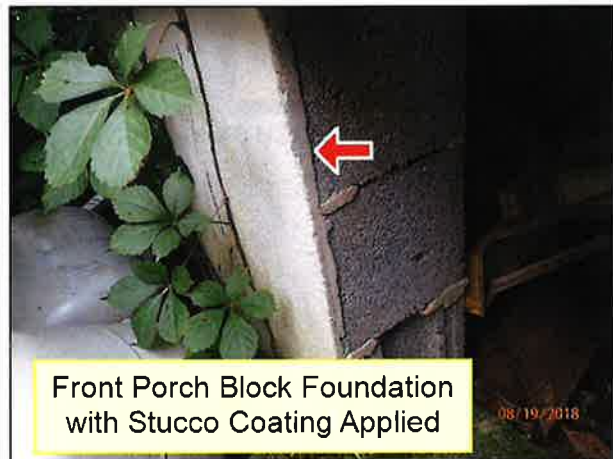
2.7 FOUNDATION SURFACE (Picture 1)
