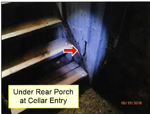
2.6 REAR PORCH (Picture 10)
