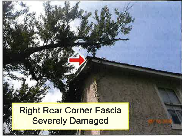
1.1 FASCIA / SOFFITS (Picture 4)
