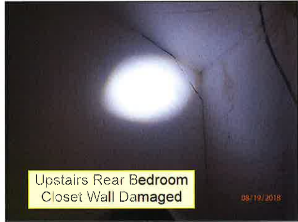
4.1 WALLS / STRUCTURE (Picture 3)
