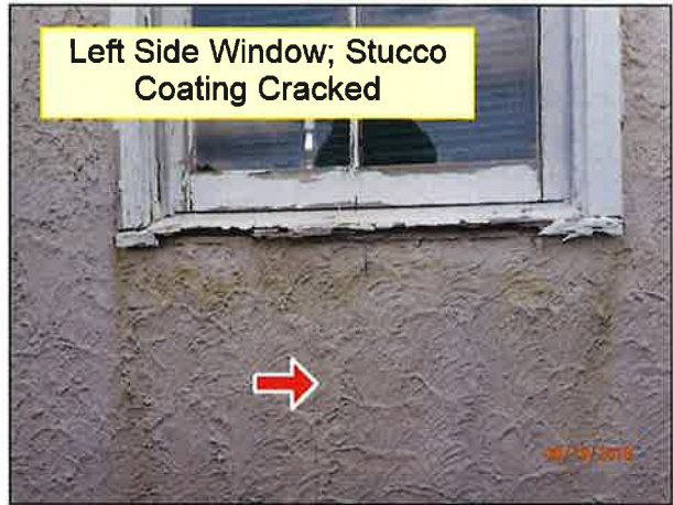
2.0 SIDING / WALL CLADDING (Picture 8)
