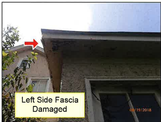
1.1 FASCIA / SOFFITS (Picture 2)
