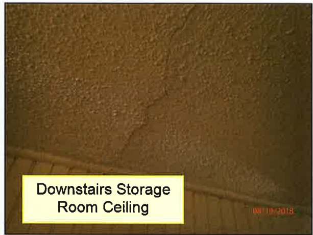
4.0 CEILINGS / STRUCTURE (Picture 10)
