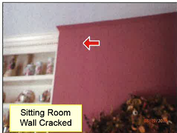
4.1 WALLS / STRUCTURE (Picture 11)
