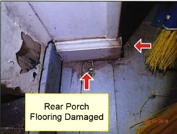
2.6 REAR PORCH (Picture 4)
