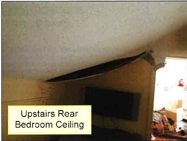
4.0 CEILINGS / STRUCTURE (Picture 3)
