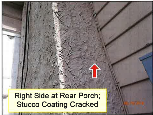
2.0 SIDING / WALL CLADDING (Picture 4)
