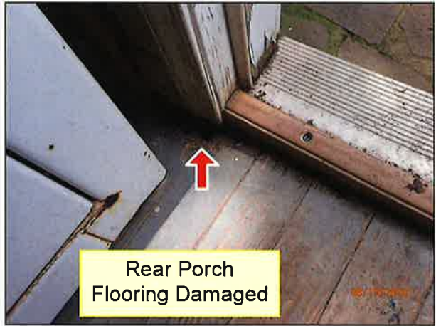
2.6 REAR PORCH (Picture 1)
