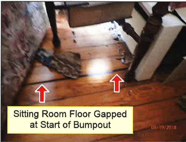
4.2 FLOORS (FRAMED) (Picture 7)
