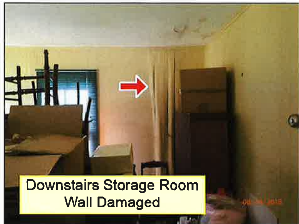
4.1 WALLS / STRUCTURE (Picture 7)
