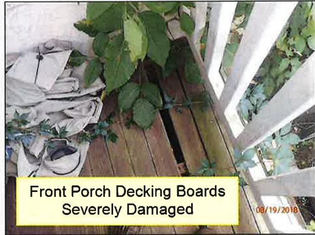
2.5 FRONT PORCH (Picture 11)
