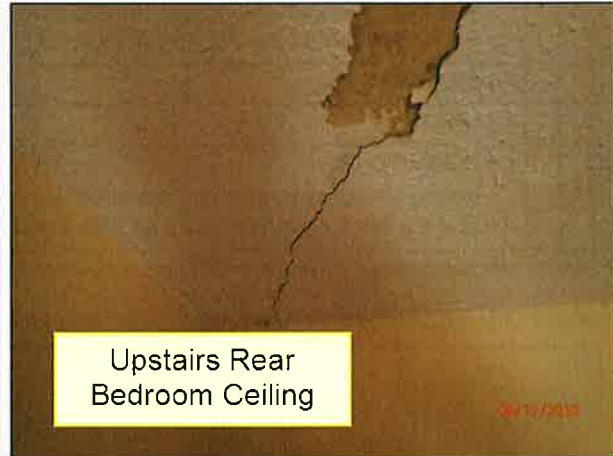
4.0 CEILINGS / STRUCTURE (Picture 8)
