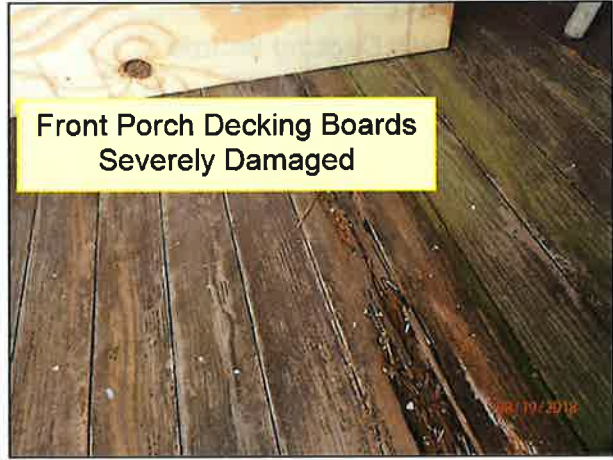
2.5 FRONT PORCH (Picture 9)
