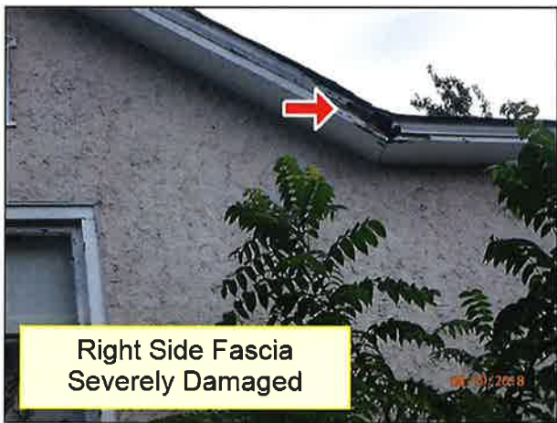
1.1 FASCIA / SOFFITS (Picture 1)
