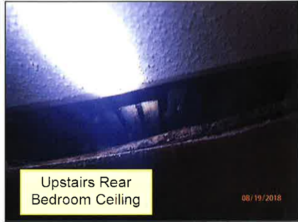
4.0 CEILINGS / STRUCTURE (Picture 6)
