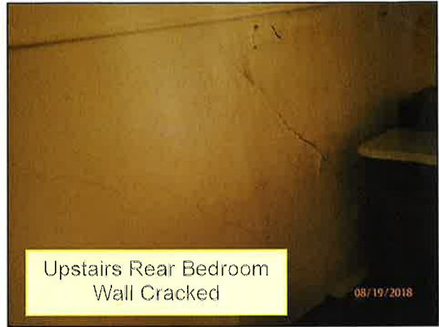
4.1 WALLS / STRUCTURE (Picture 1)
