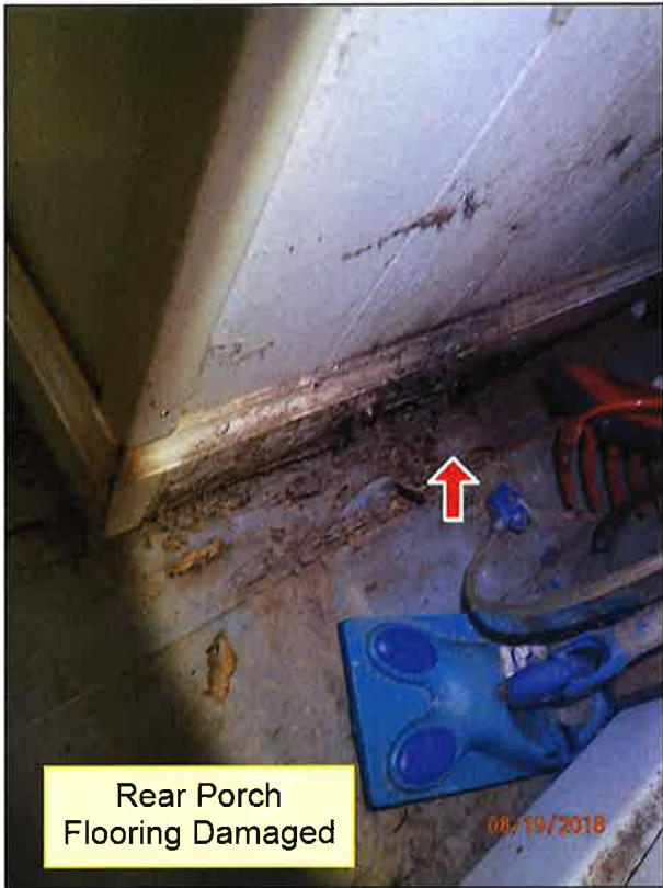
2.6 REAR PORCH (Picture 6)
