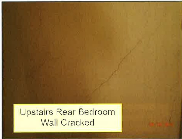
4.1 WALLS / STRUCTURE (Picture 2)
