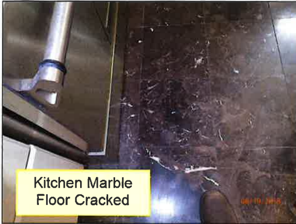
4.2 FLOORS (FRAMED) (Picture 5)
