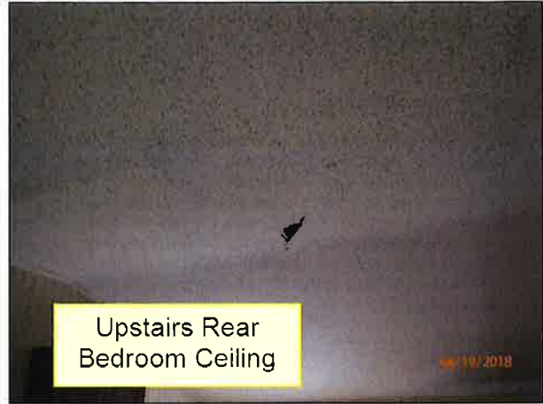
4.0 CEILINGS / STRUCTURE (Picture 4)
