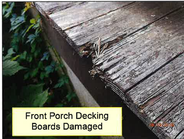
2.5 FRONT PORCH (Picture 10)
