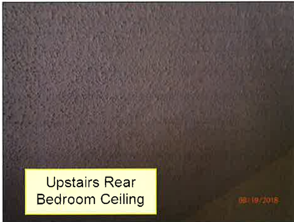
4.0 CEILINGS / STRUCTURE (Picture 7)
