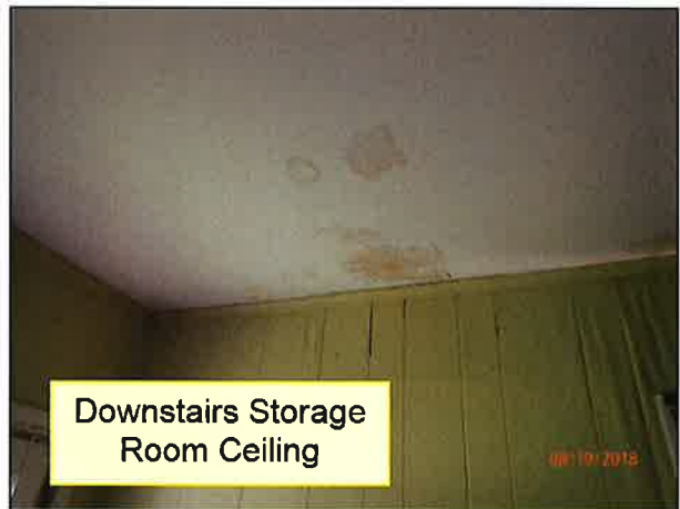
4.0 CEILINGS / STRUCTURE (Picture 12)
