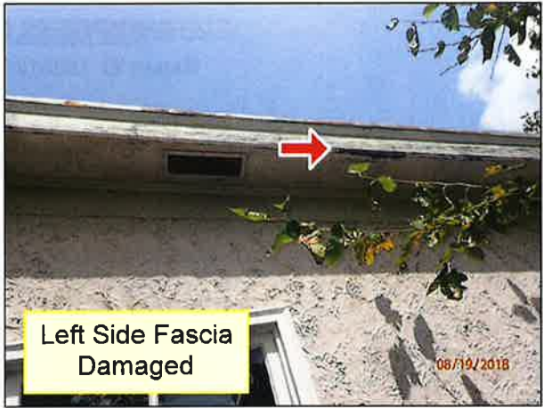
1.1 FASCIA / SOFFITS (Picture 3)
