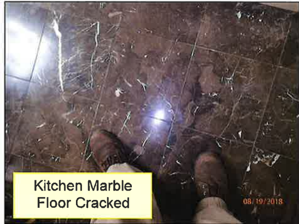
4.2 FLOORS (FRAMED) (Picture 6)
