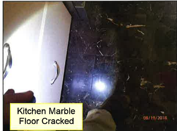
4.2 FLOORS (FRAMED) (Picture 4)
