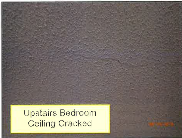
4.0 CEILINGS / STRUCTURE (Picture 15)
