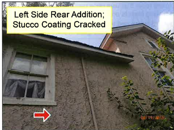
2.0 SIDING / WALL CLADDING (Picture 5)
