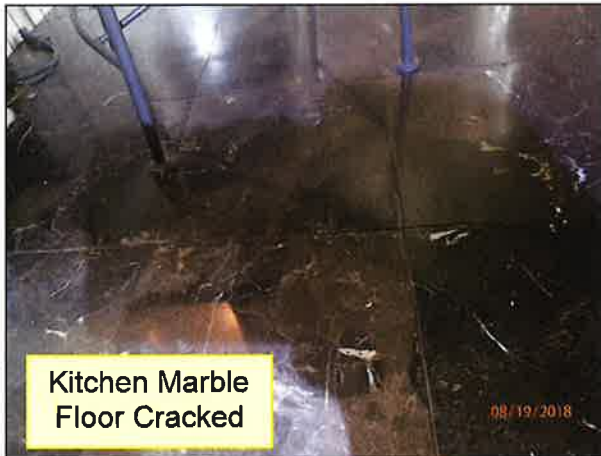
4.2 FLOORS (FRAMED) (Picture 3)
