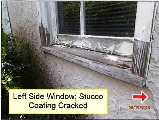
2.0 SIDING / WALL CLADDING (Picture 7)
