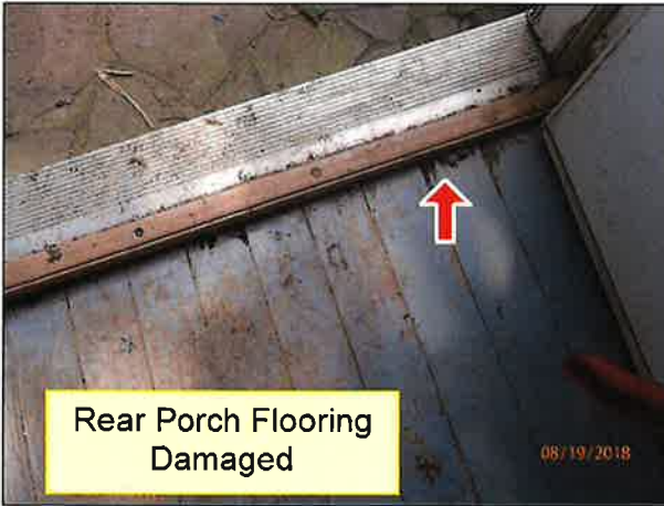
2.6 REAR PORCH (Picture 2)
