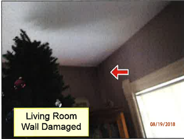
4.1 WALLS / STRUCTURE (Picture 12)
