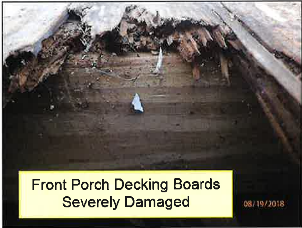
2.5 FRONT PORCH (Picture 6)
