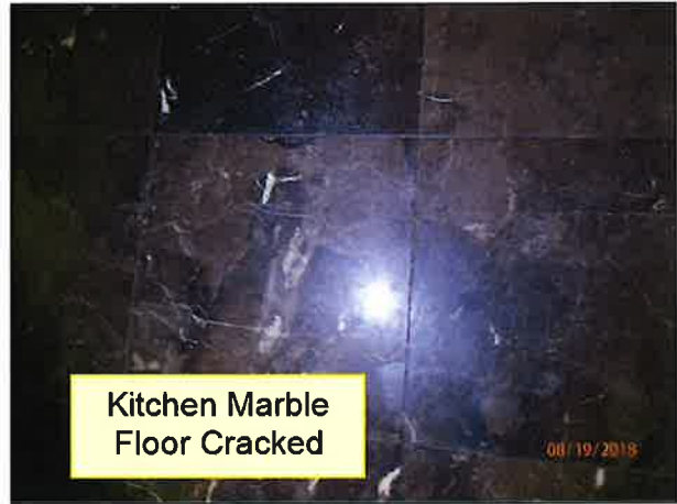
4.2 FLOORS (FRAMED) (Picture 2)
