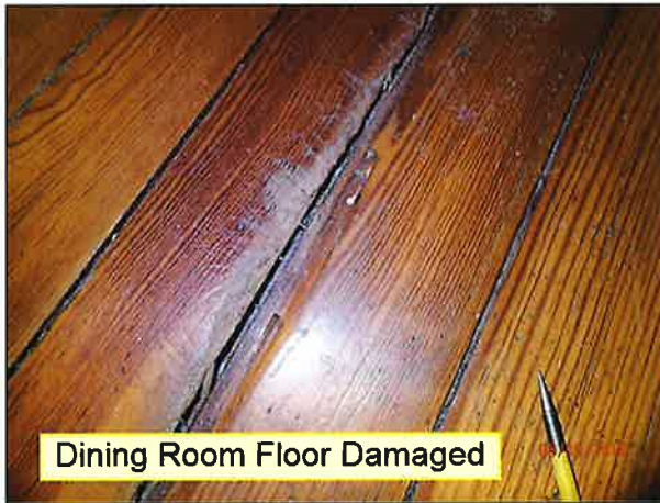
4.2 FLOORS (FRAMED) (Picture 1)
