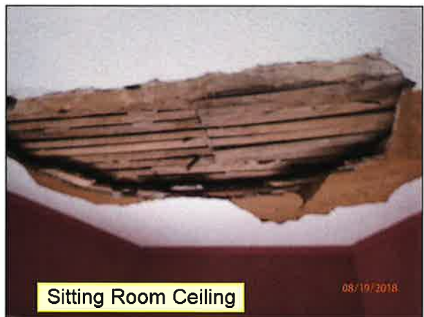
4.0 CEILINGS / STRUCTURE (Picture 14)
