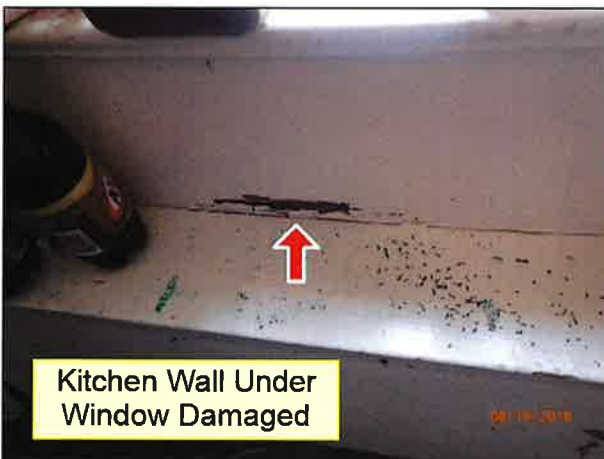
4.1 WALLS / STRUCTURE (Picture 10)
