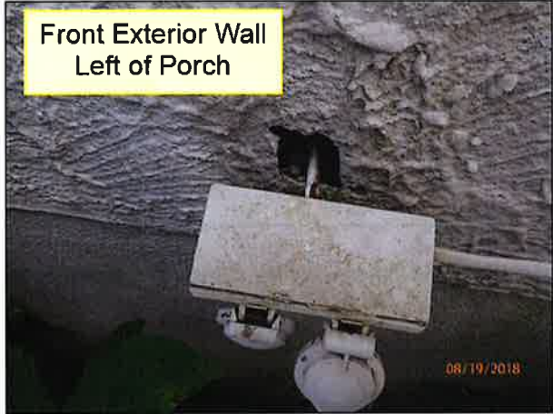
2.0 SIDING / WALL CLADDING (Picture 1)
