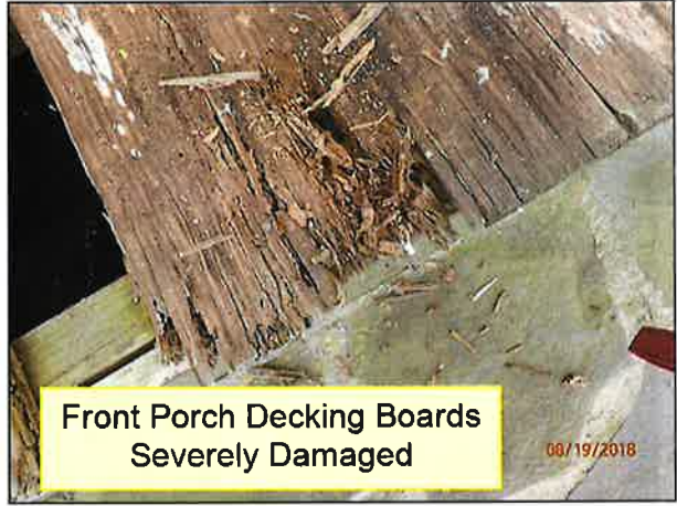
2.5 FRONT PORCH (Picture 7)
