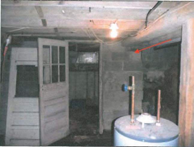
Photo 4 – View of foundation showing some settlement and dirt crawl space Photo 5– View of foundation showing settlement crack at corner.
