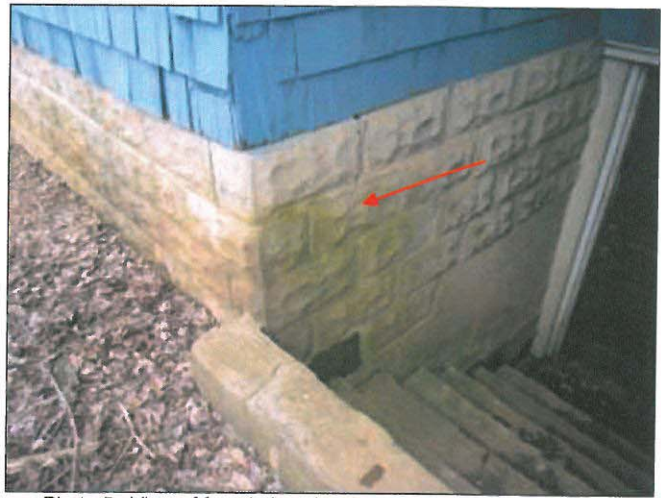
Photo 4 – View of foundation showing some settlement and dirt crawl space Photo 5– View of foundation showing settlement crack at corner.
