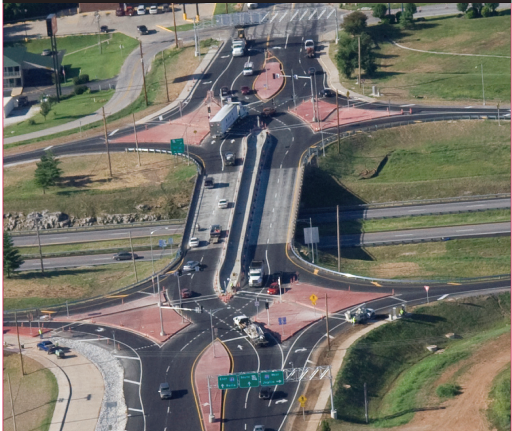
Figure 1. First U.S. DCD interchange at I-44 and Route 13 in Springfield, MO.
