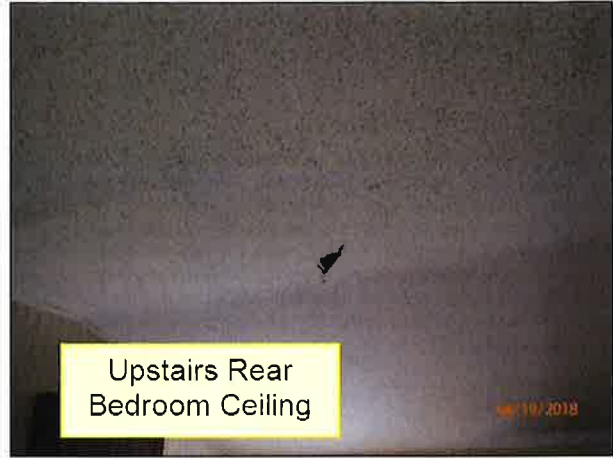
4.0 CEILINGS / STRUCTURE (Picture 4)
