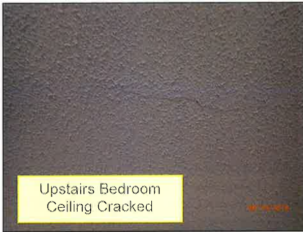
4.0 CEILINGS / STRUCTURE (Picture 15)
