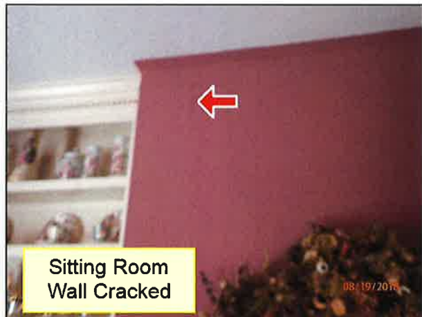
4.1 WALLS / STRUCTURE (Picture 11)
