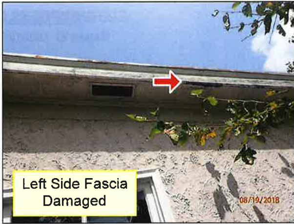
1.1 FASCIA / SOFFITS (Picture 3)
