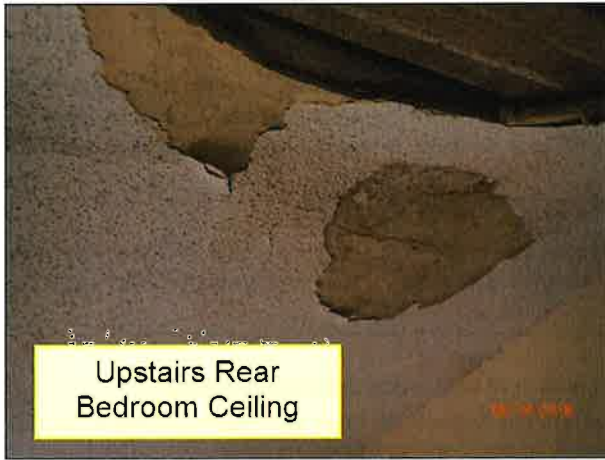
4.0 CEILINGS / STRUCTURE (Picture 5)
