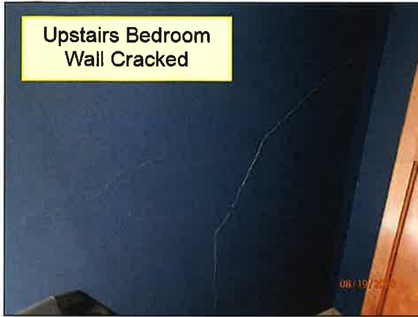
4.1 WALLS / STRUCTURE (Picture 6)
