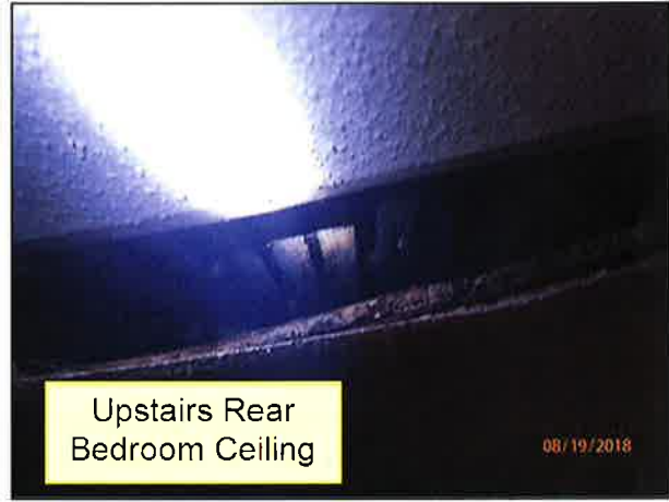
4.0 CEILINGS / STRUCTURE (Picture 6)
