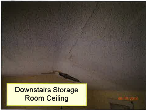
4.0 CEILINGS / STRUCTURE (Picture 9)
