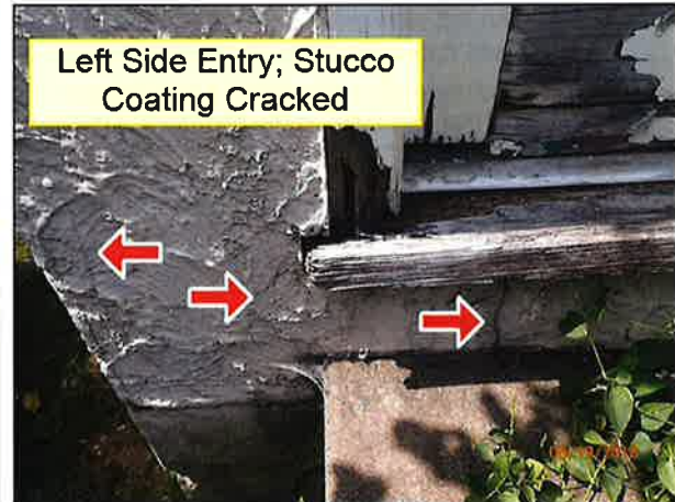
2.0 SIDING / WALL CLADDING (Picture 6)
