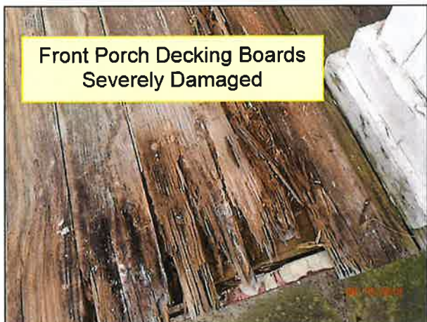
2.5 FRONT PORCH (Picture 8)
