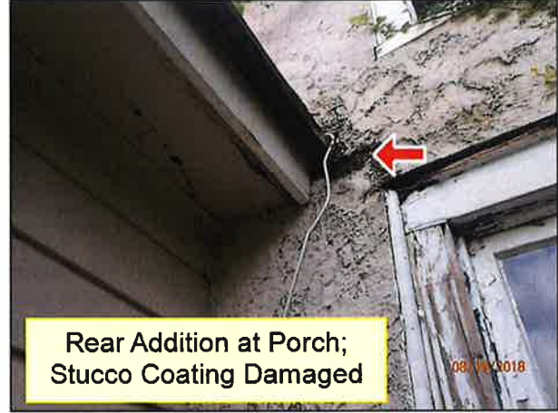
2.0 SIDING / WALL CLADDING (Picture 2)
