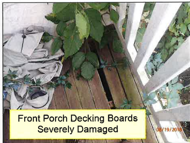
2.5 FRONT PORCH (Picture 11)
