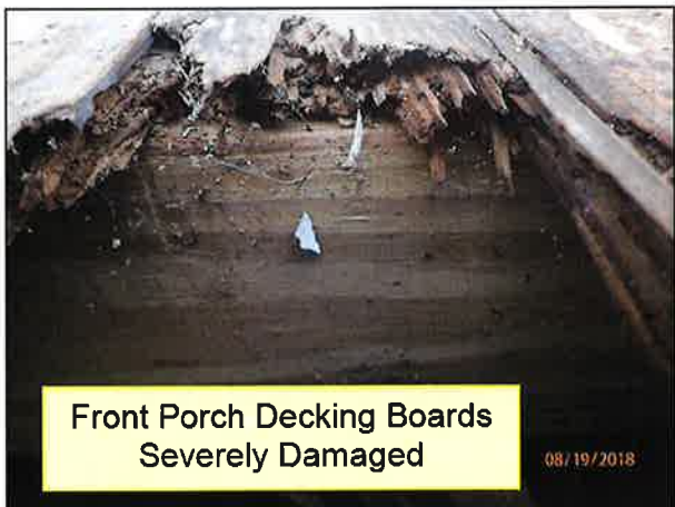
2.5 FRONT PORCH (Picture 6)
