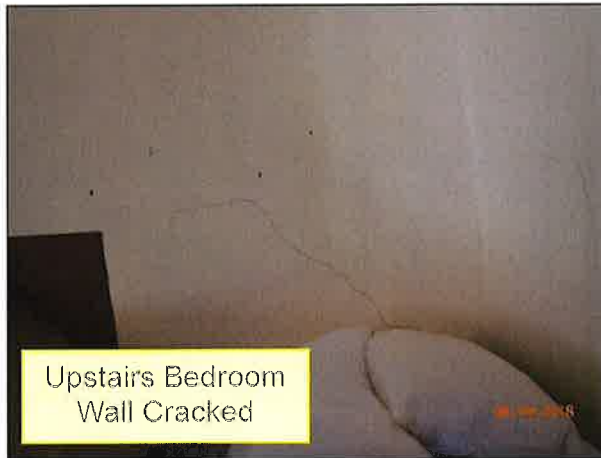
4.1 WALLS / STRUCTURE (Picture 4)
