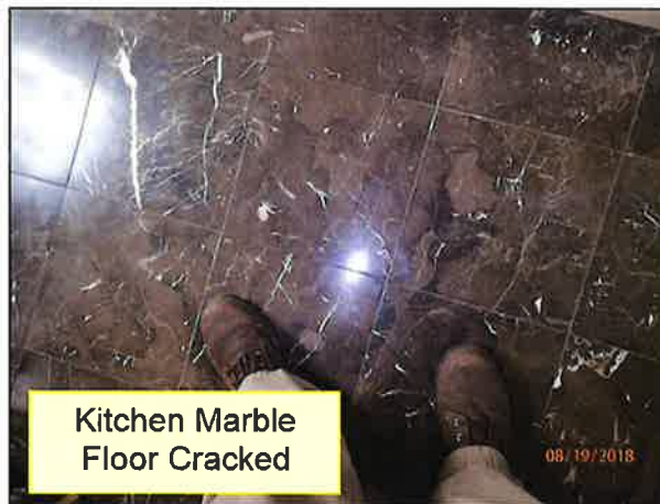
4.2 FLOORS (FRAMED) (Picture 6)
