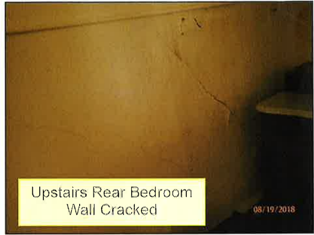
4.1 WALLS / STRUCTURE (Picture 1)
