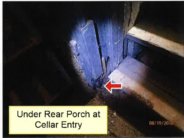
2.6 REAR PORCH (Picture 9)
