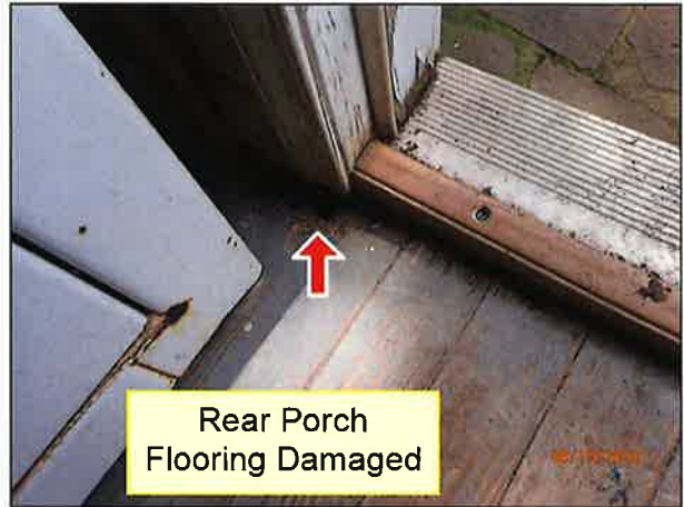
2.6 REAR PORCH (Picture 1)
