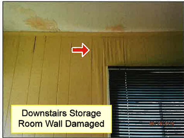
4.1 WALLS / STRUCTURE (Picture 9)
