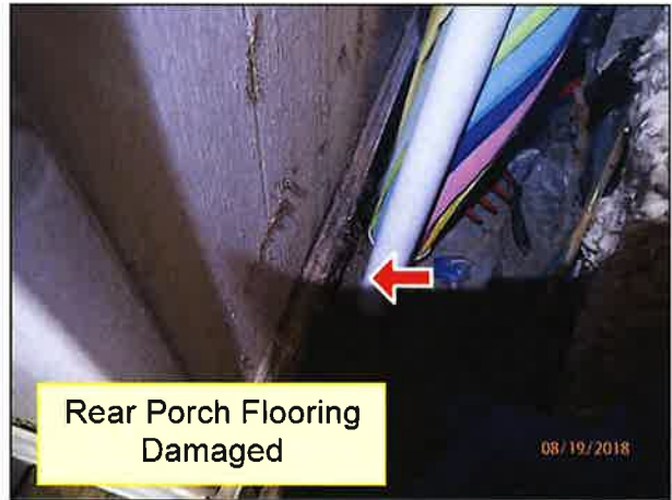
2.6 REAR PORCH (Picture 3)
