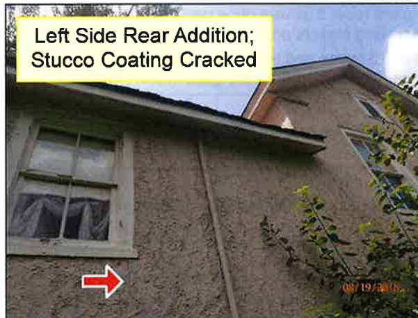
2.0 SIDING / WALL CLADDING (Picture 5)
