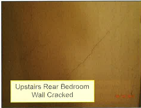
4.1 WALLS / STRUCTURE (Picture 2)
