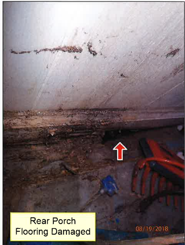
2.6 REAR PORCH (Picture 5)
