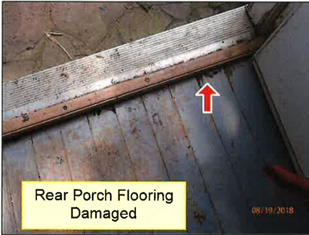
2.6 REAR PORCH (Picture 2)
