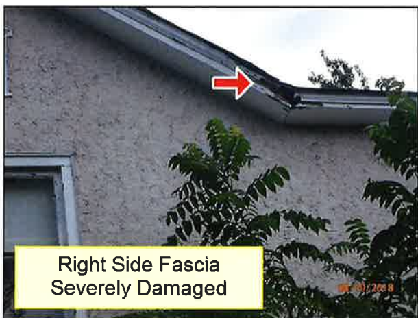
1.1 FASCIA / SOFFITS (Picture 1)
