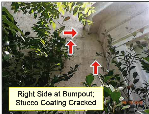
2.0 SIDING / WALL CLADDING (Picture 3)
