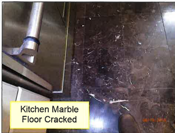
4.2 FLOORS (FRAMED) (Picture 5)
