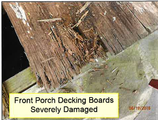
2.5 FRONT PORCH (Picture 7)
