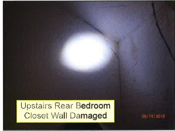
4.1 WALLS / STRUCTURE (Picture 3)
