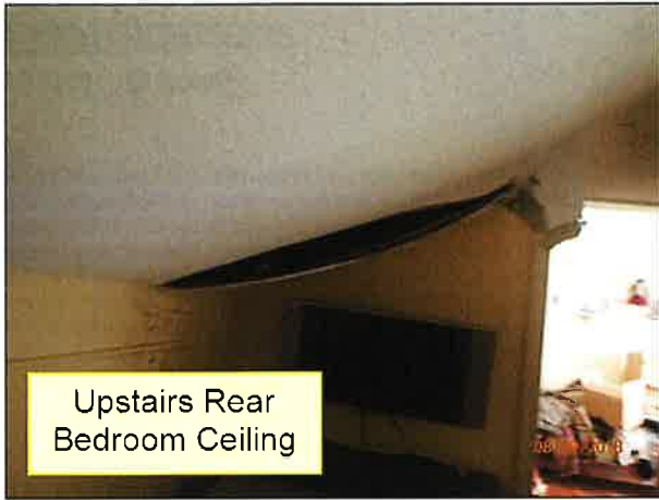
4.0 CEILINGS / STRUCTURE (Picture 3)
