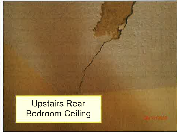
4.0 CEILINGS / STRUCTURE (Picture 8)
