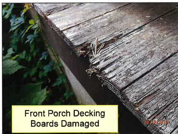
2.5 FRONT PORCH (Picture 10)
