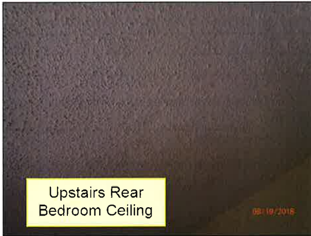
4.0 CEILINGS / STRUCTURE (Picture 7)
