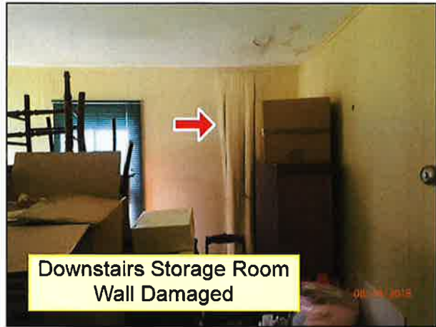
4.1 WALLS / STRUCTURE (Picture 7)
