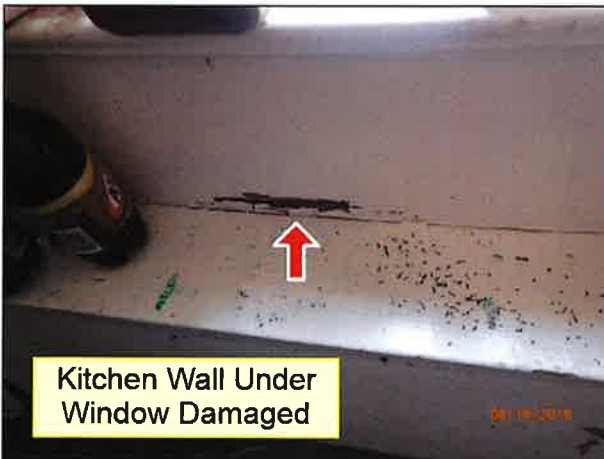
4.1 WALLS / STRUCTURE (Picture 10)
