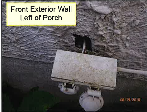
2.0 SIDING / WALL CLADDING (Picture 1)
