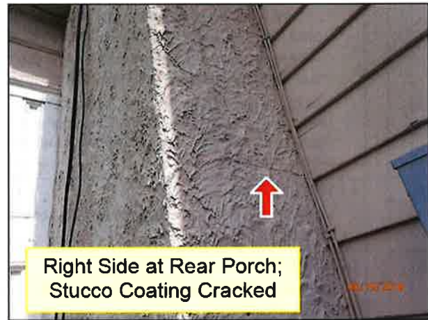
2.0 SIDING / WALL CLADDING (Picture 4)
