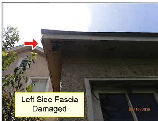
1.1 FASCIA / SOFFITS (Picture 2)
