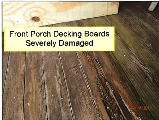
2.5 FRONT PORCH (Picture 9)
