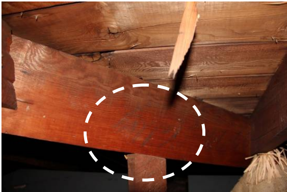
Grease handwritten numbers in attic of 14710, an indicator of a Lewis Manufacturing-made home.
