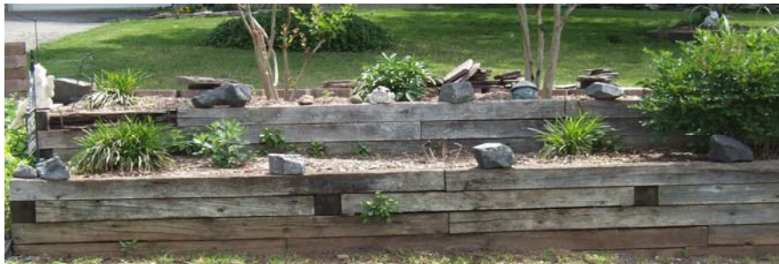
Wood Retaining Wall
