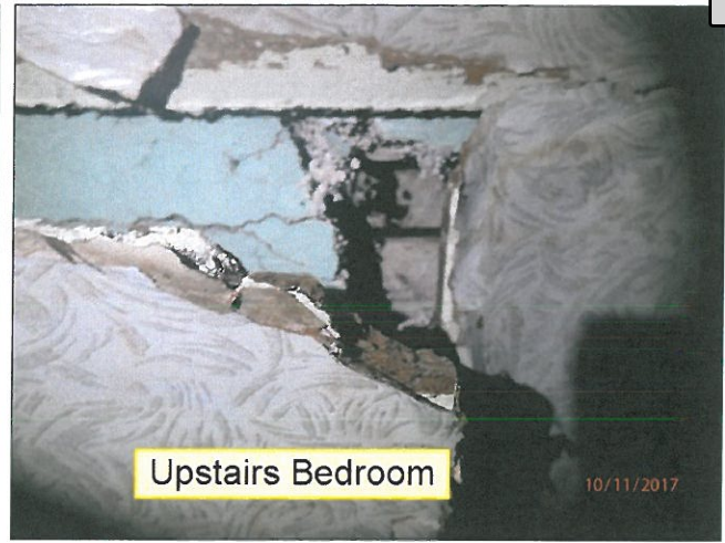
4.0 CEILINGS / STRUCTURE (Picture 2)
