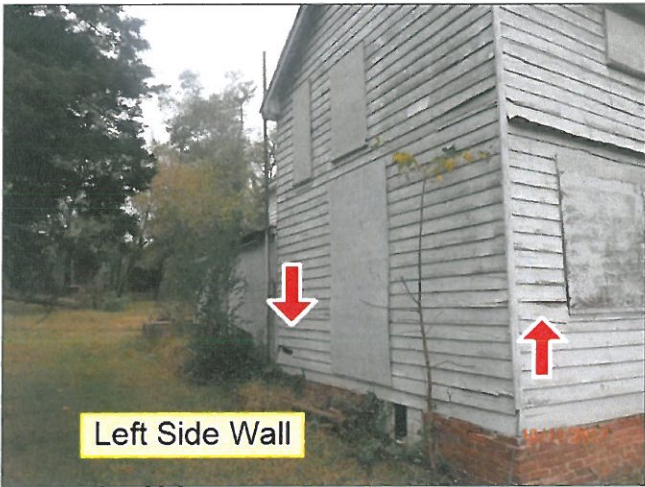
2.0 SIDING / WALL CLADDING (Picture 5)
