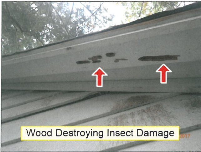
1.6 FASCIA / SOFFITS (Picture 3)
