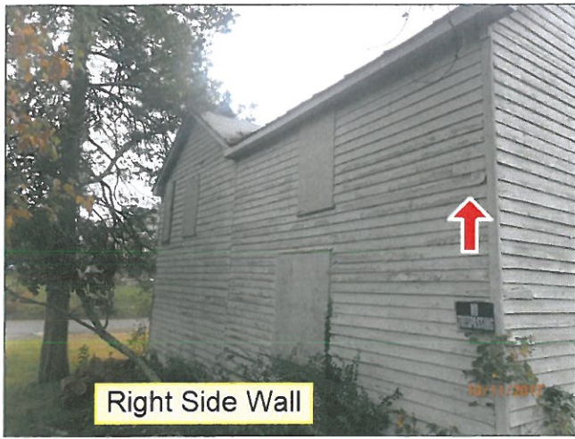
2.0 SIDING / WALL CLADDING (Picture 3)
