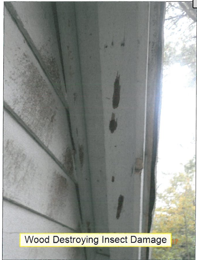
1.6 FASCIA / SOFFITS (Picture 2)
