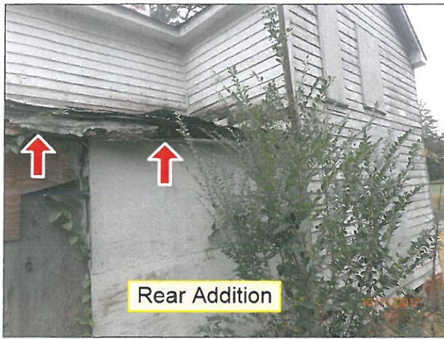
1.6 FASCIA / SOFFITS (Picture 5)
