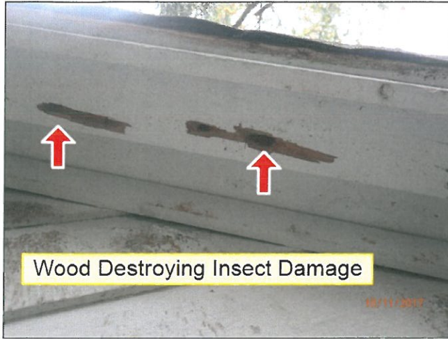
1.6 FASCIA / SOFFITS (Picture 1)
