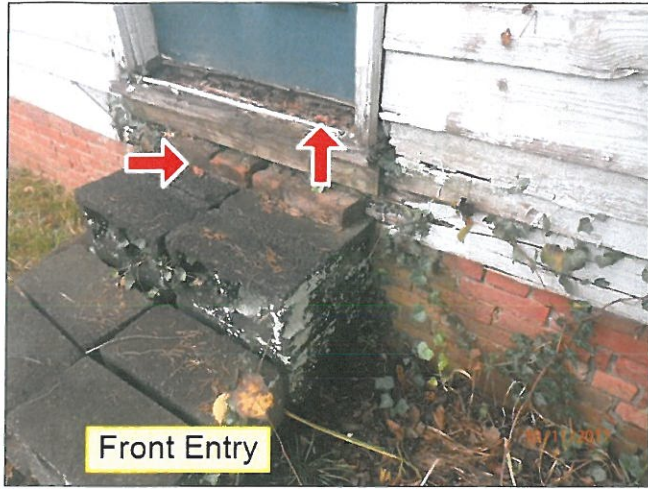
2.2 ENTRY DOORS (Picture 1)
