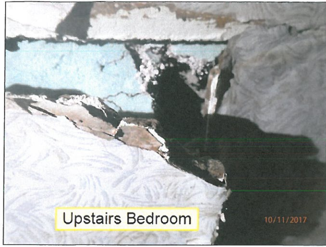
4.0 CEILINGS / STRUCTURE (Picture 1)
