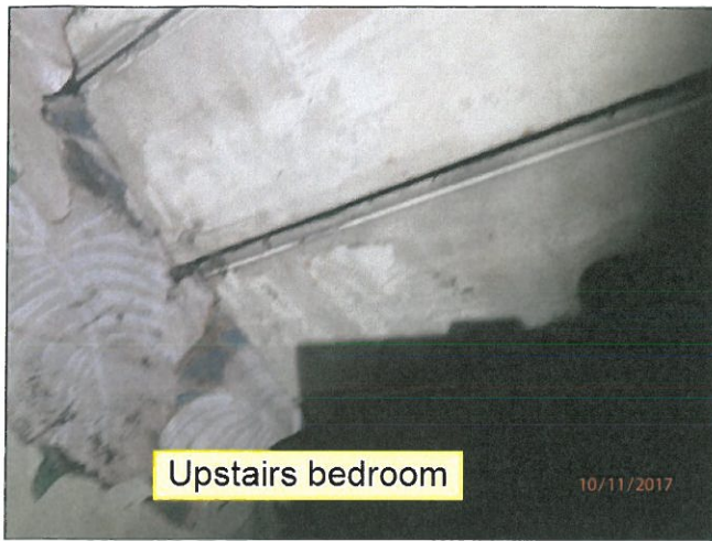
4.0 CEILINGS / STRUCTURE (Picture 7)
