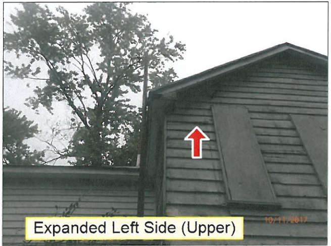
2.0 SIDING / WALL CLADDING (Picture 8)
