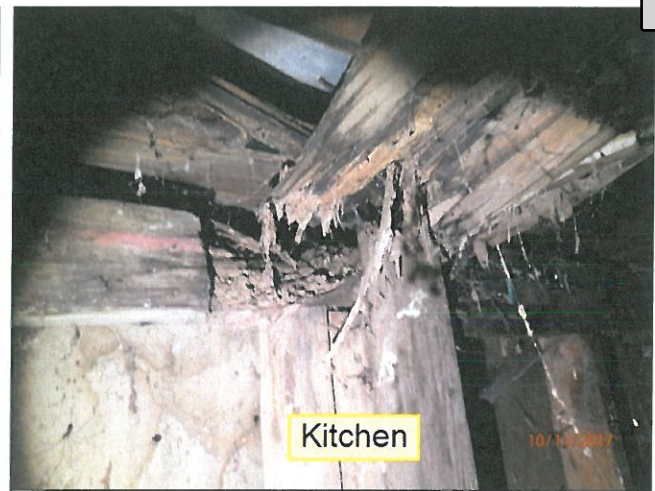
4.0 CEILINGS / STRUCTURE (Picture 8)
