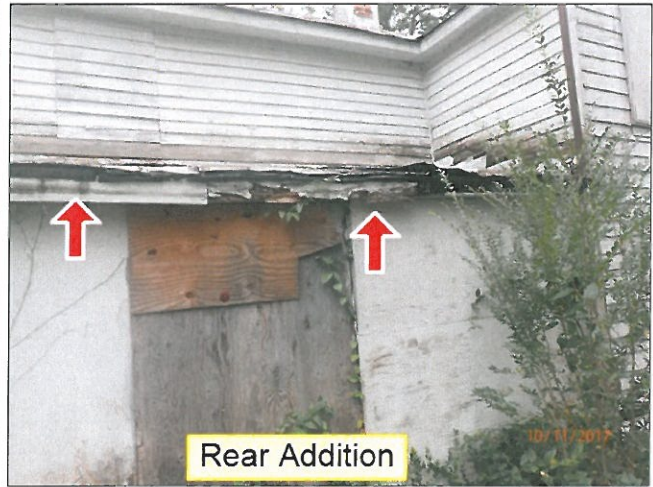
1.6 FASCIA / SOFFITS (Picture 4)
