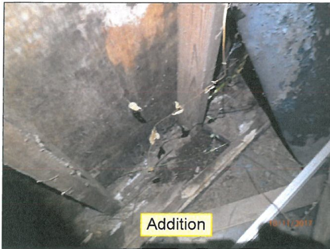
4.0 CEILINGS / STRUCTURE (Picture 9)
