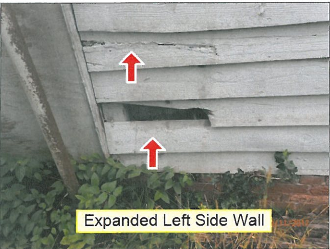
2.0 SIDING / WALL CLADDING (Picture 7)
