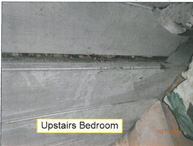
4.0 CEILINGS / STRUCTURE (Picture 5)
