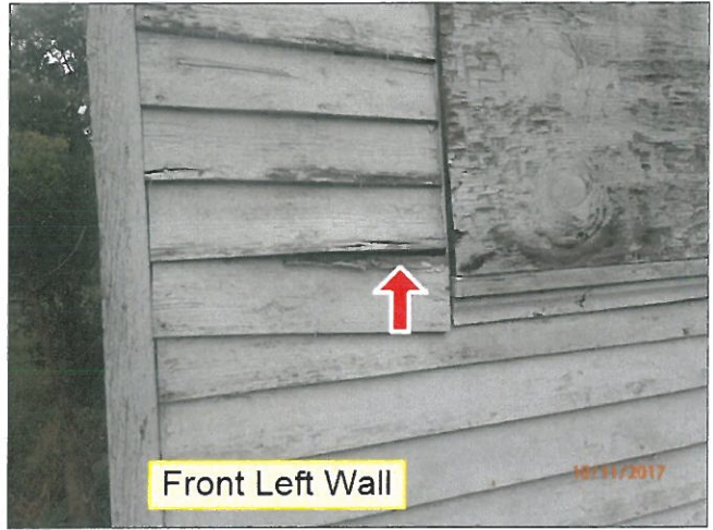
2.0 SIDING / WALL CLADDING (Picture 6)
