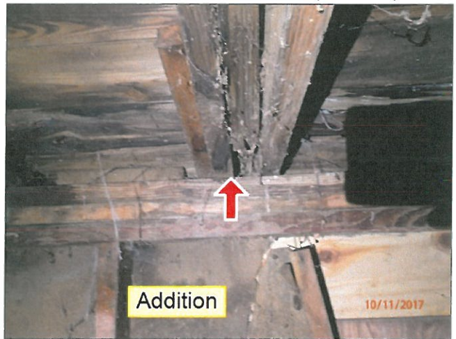
4.0 CEILINGS / STRUCTURE (Picture 10)
