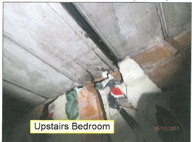
4.0 CEILINGS / STRUCTURE (Picture 6)
