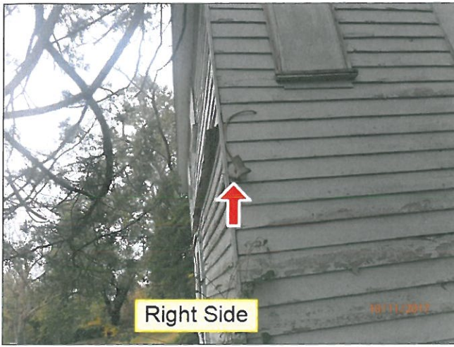
2.6 ELECTRICAL / GFCI (Picture 3)
