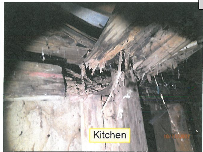
4.0 CEILINGS / STRUCTURE (Picture 8)
