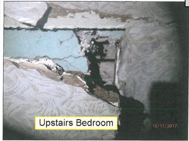
4.0 CEILINGS / STRUCTURE (Picture 2)
