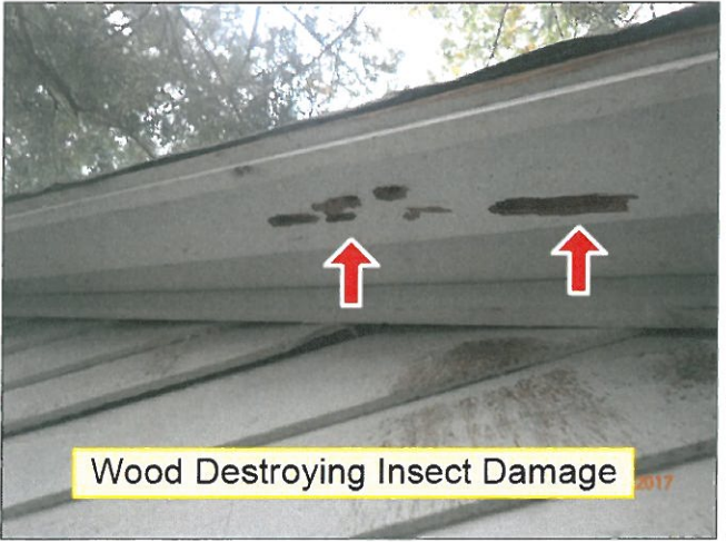
1.6 FASCIA / SOFFITS (Picture 3)
