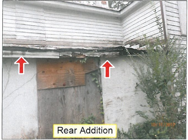
1.6 FASCIA / SOFFITS (Picture 4)
