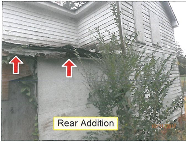
1.6 FASCIA / SOFFITS (Picture 5)
