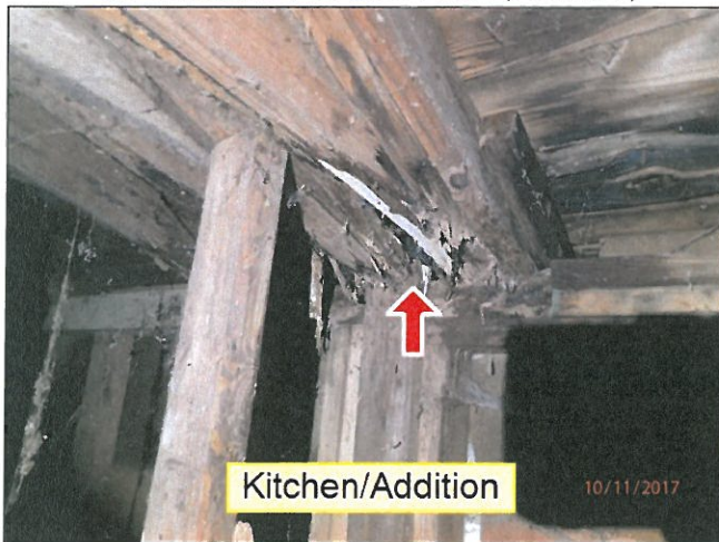
4.0 CEILINGS / STRUCTURE (Picture 11)
