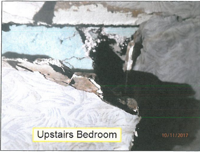
4.0 CEILINGS / STRUCTURE (Picture 1)
