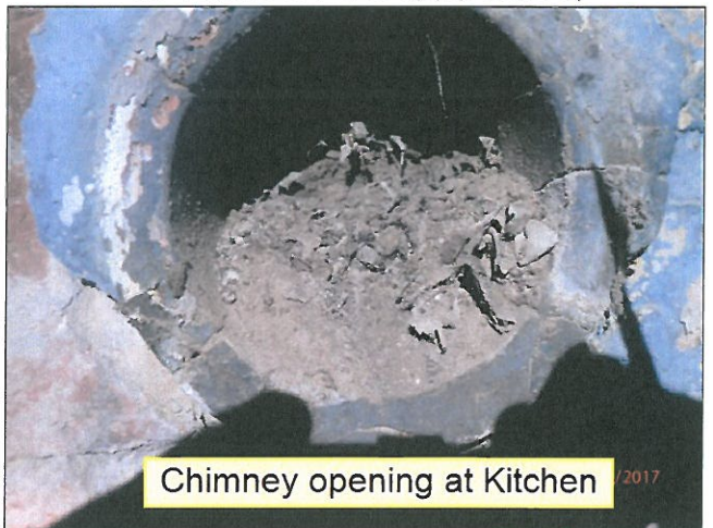
1.3 CHIMNEY / VENT(s) (Picture 5)
