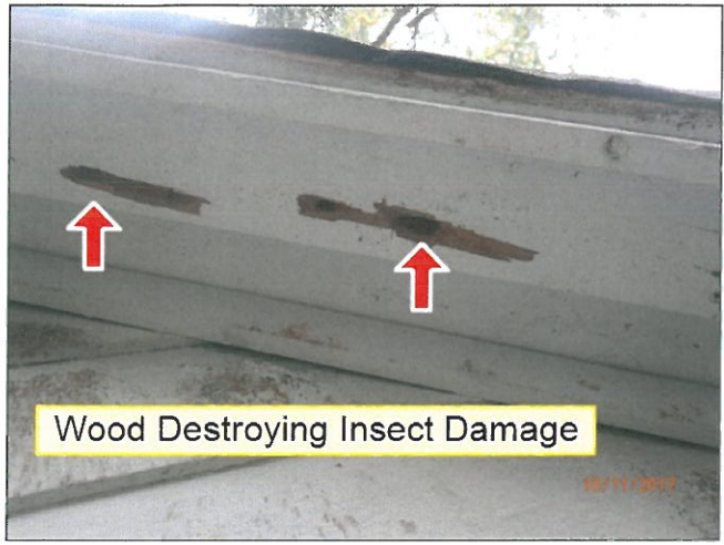
1.6 FASCIA / SOFFITS (Picture 1)
