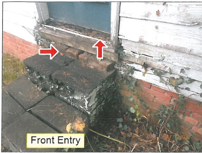
2.2 ENTRY DOORS (Picture 1)
