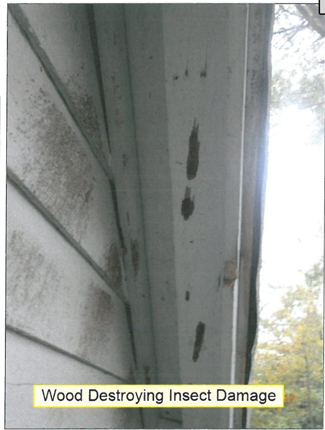
1.6 FASCIA / SOFFITS (Picture 2)
