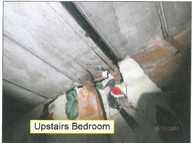
4.0 CEILINGS / STRUCTURE (Picture 6)
