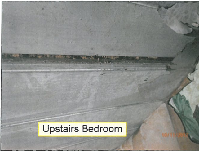
4.0 CEILINGS / STRUCTURE (Picture 5)
