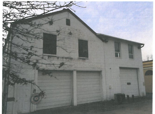
Photo 13 – North elevations – Front at Washington St
