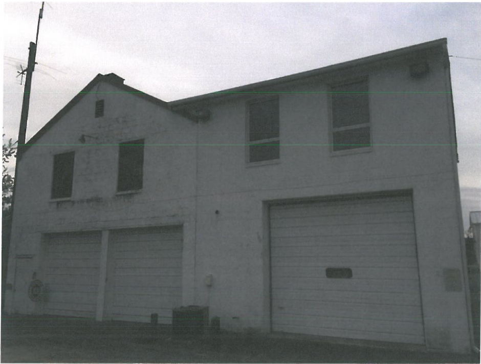
Photo 1 – View from Washington Street
