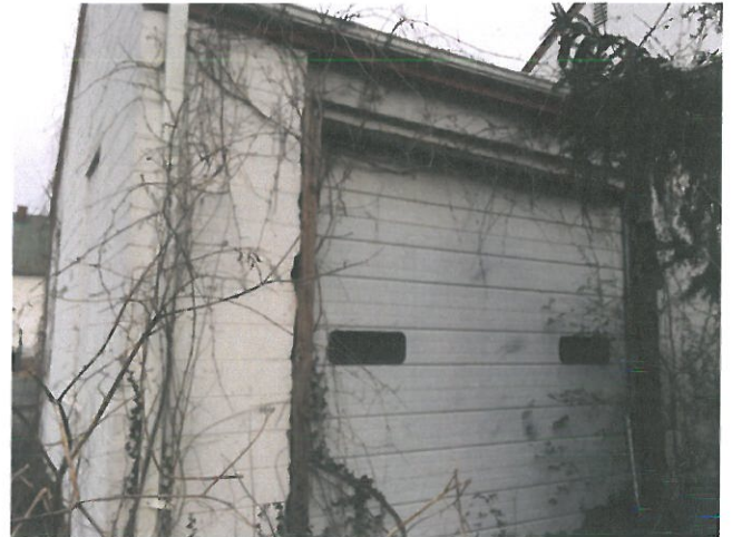
Photo 15 – Southeast Corner (rear)
