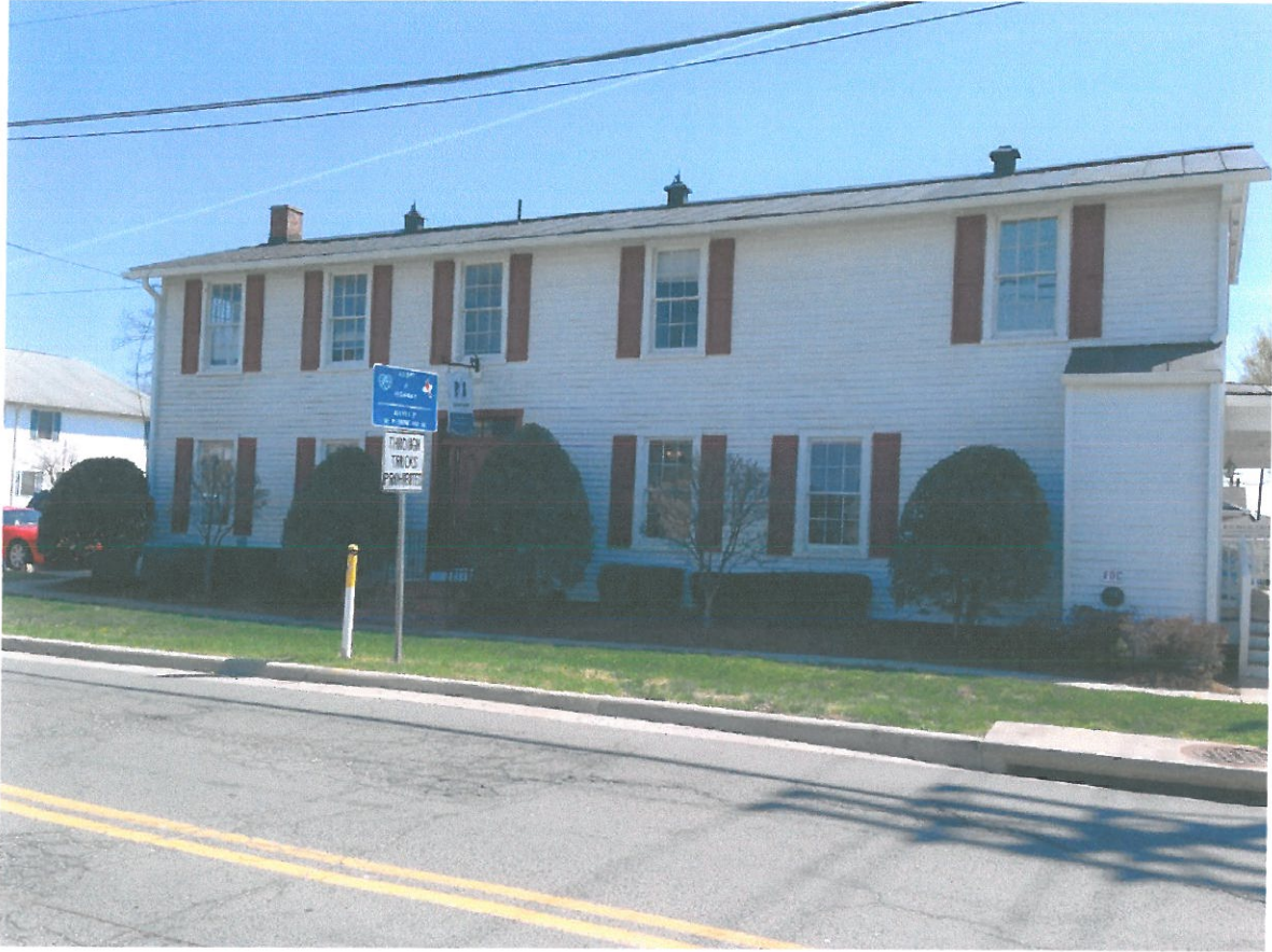
14950 WASHINGTON STREET (VIEW FROM JEFFERSON STREET)
