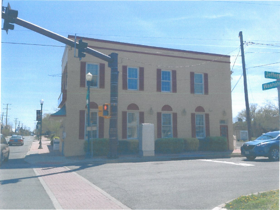
14951 WASHINGTON STREET (VIEW FROM JEFFERSON STREET)
