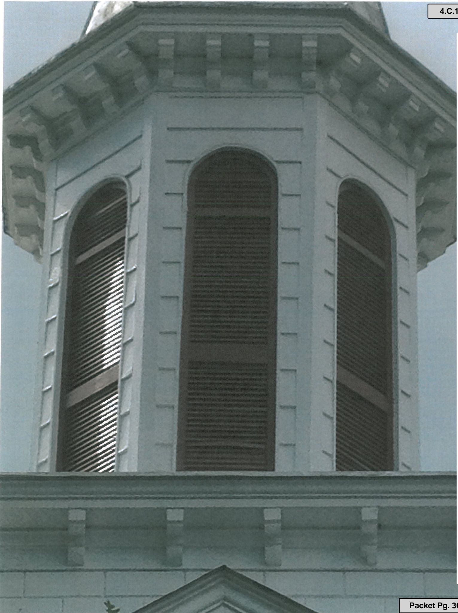
Attachment: 6760 Fayette Street - Shutter Replacement (2359 : 6760 Fayette Street - Shutter Replacement)
