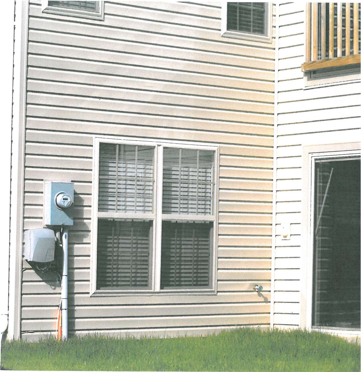
Attachment: 14723 Alexandras Keep Lane - Deck (AGI-2014-99 : 14723 Alexandra's Keep Lane)
