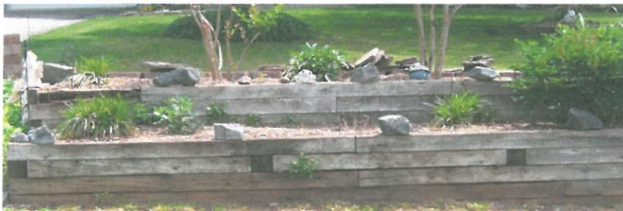
Wood Retaining Wall
