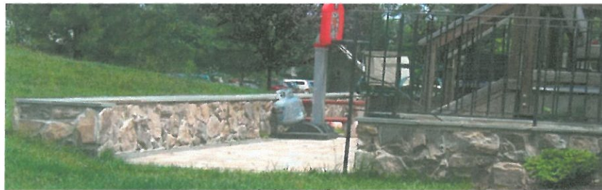
Stone Retaining Wall
