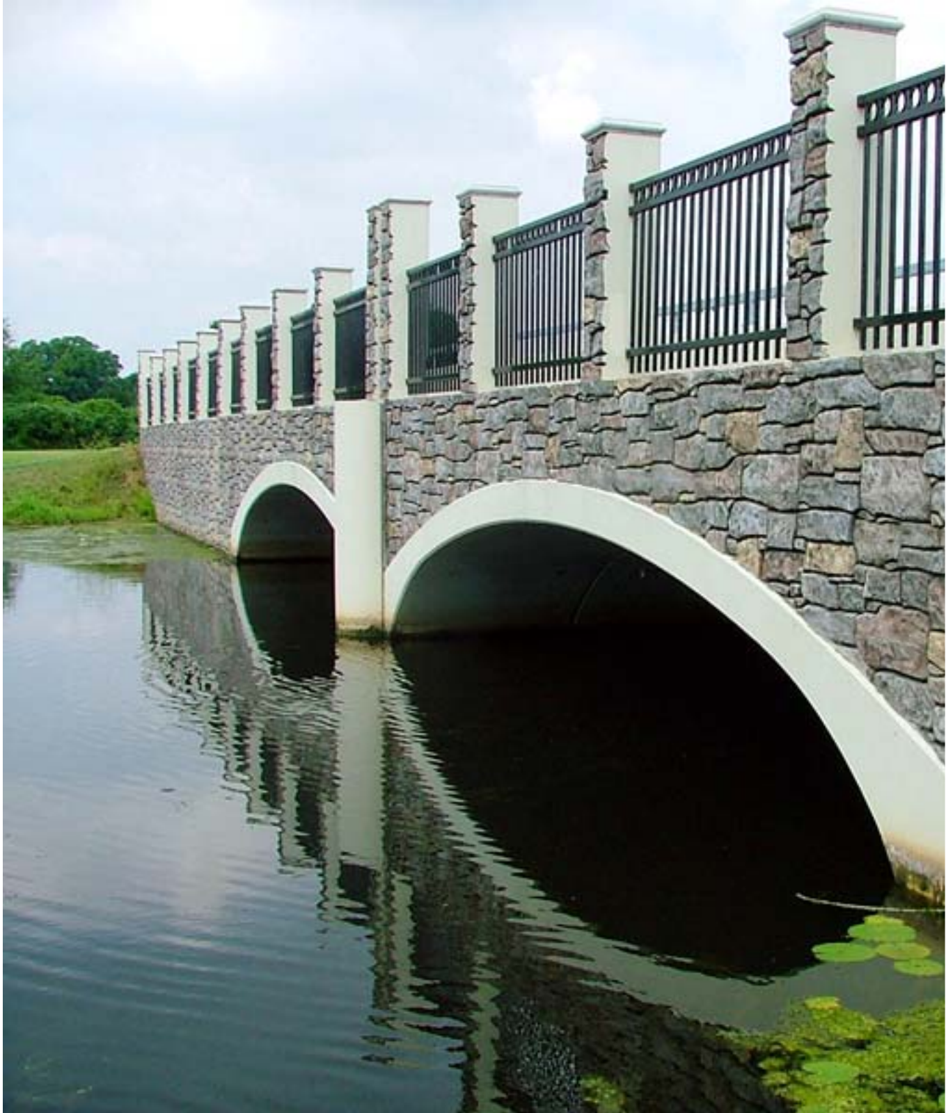
A sample of staining form lined bridge facade.
