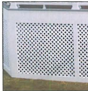
WHITE PVC LATTICE AROUND PERIMETER BELOW BOTH DECKS
