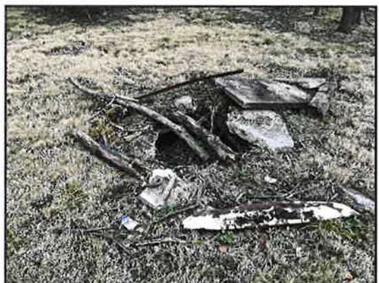
PHOTO 6: In-Ground Concrete Structure
