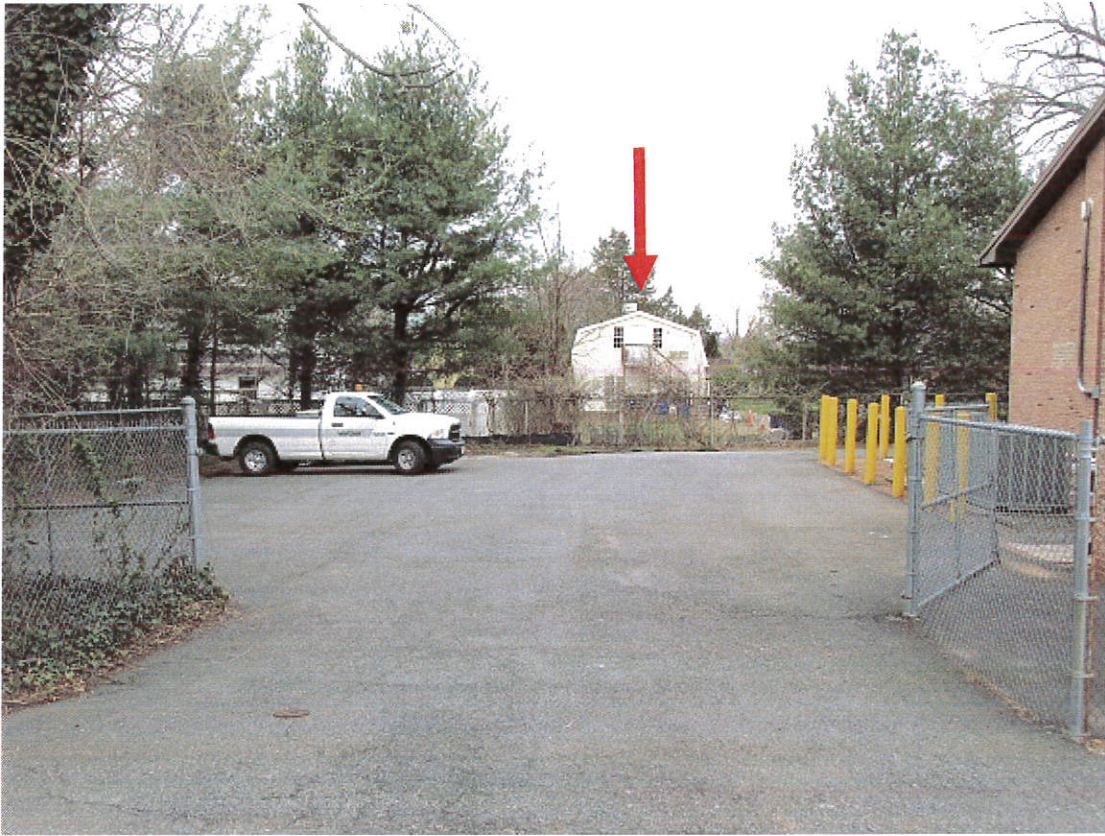
CLOSEST NEIGHBORING STRUCTURE
