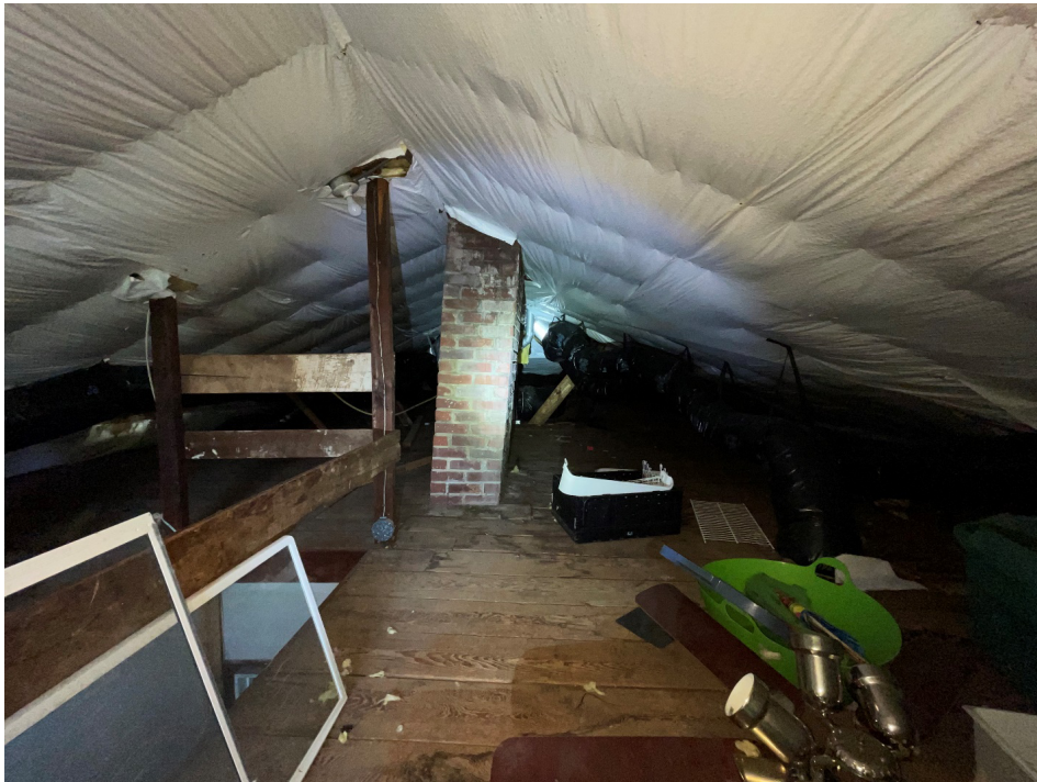
Attic Observation #1 thru #3
