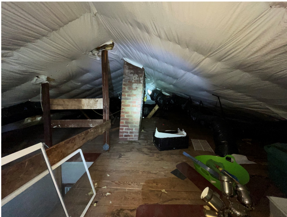
Attic Observation #1 thru #3
