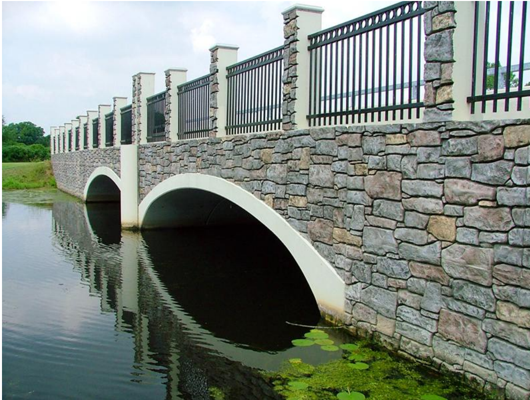
The color treatment technique on the bridges will be similar to this but the colors, façade pattern and bridge design will not necessarily be the same.
