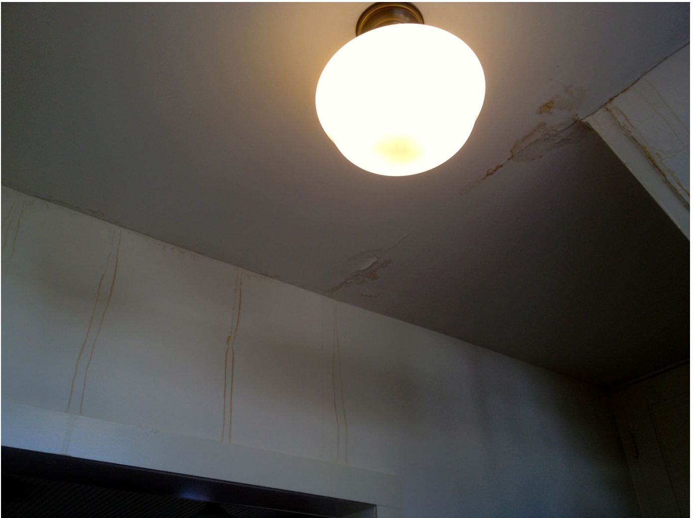
1 st floor entryway.
