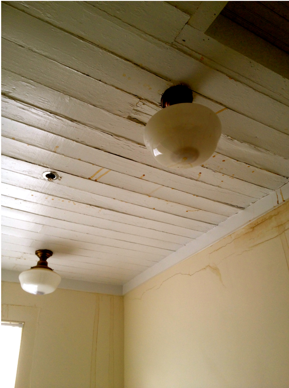
SECOND FLOOR STAIRWAY AREA
